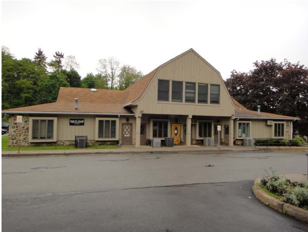
Image of existing commercial building
