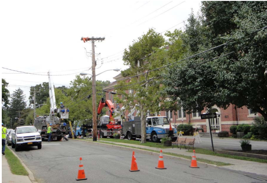
Con Edison repair crew at Municipal replacing primary service cables and transformer
