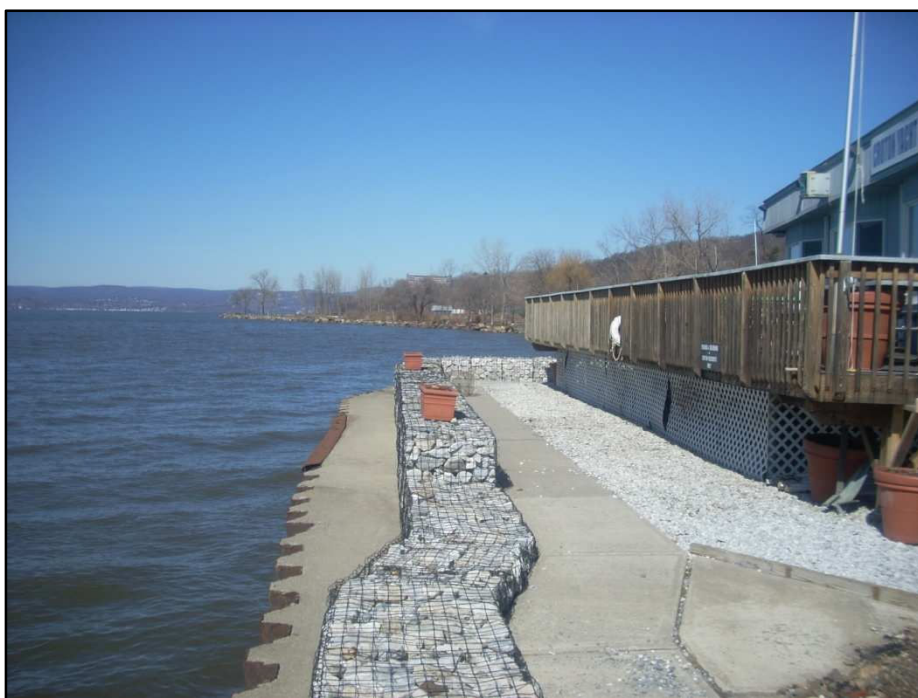
Photo 2- Shoreline Segment B "Southwest Building Area"
