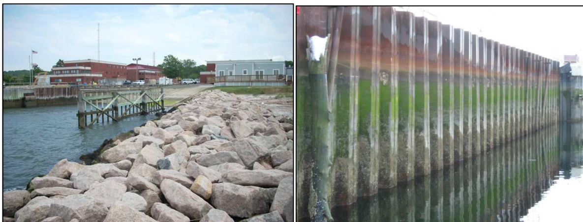
Photo 5 - Stone Revetment (left) and Cantilever Bulkhead (right)
