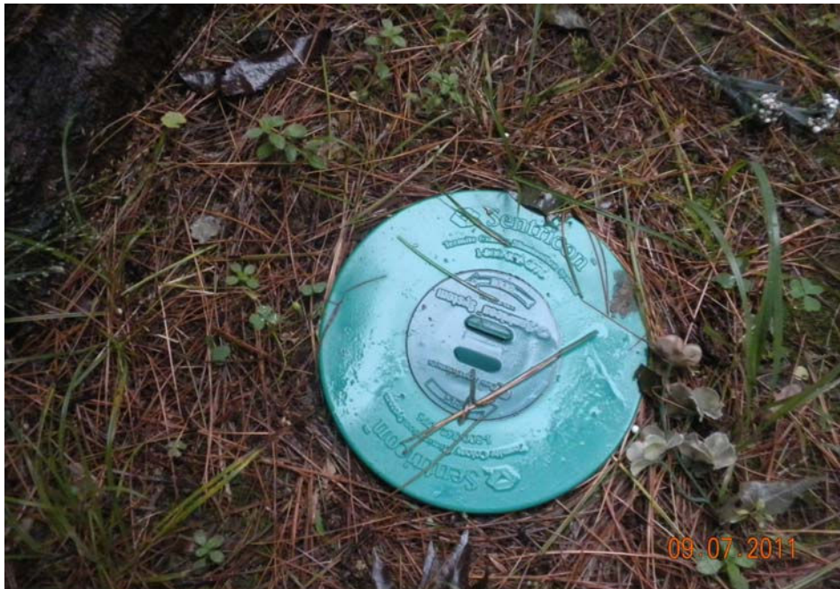
Termite treatment at perimeter of main house
