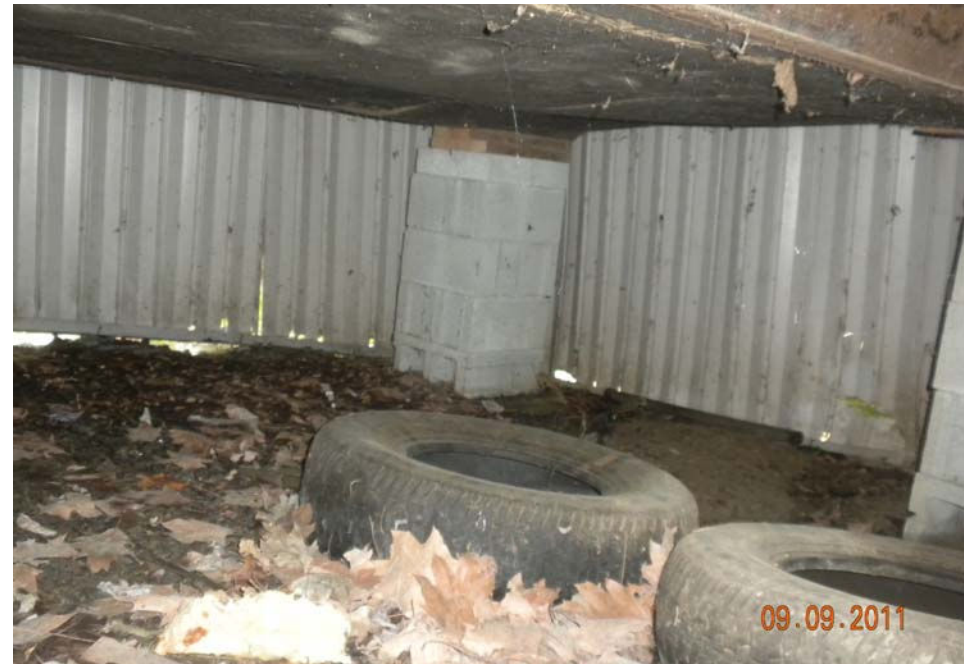
Crawl Space under Mobile Home
