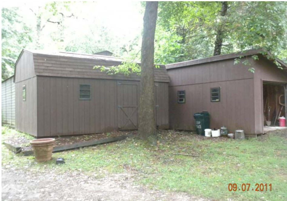
Shed/Office and one car garage
