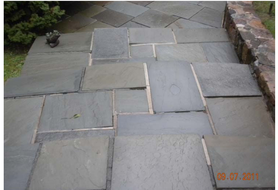
Reset uneven flags at entry walk
