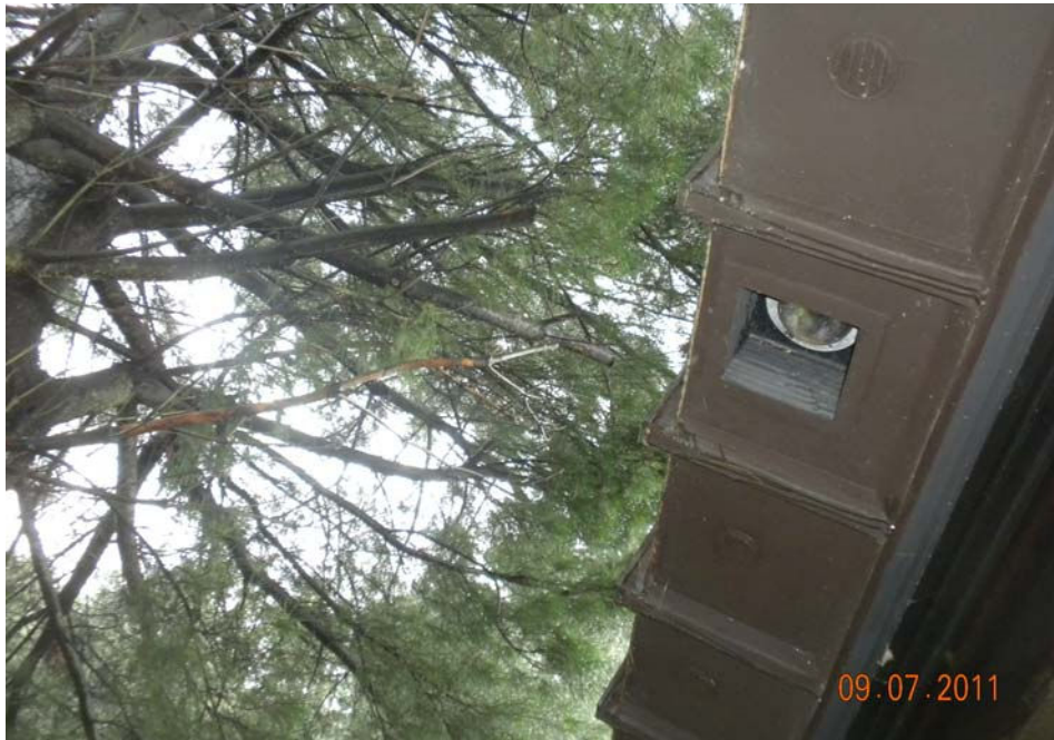
Trim back tree limbs overhanging main house roof
