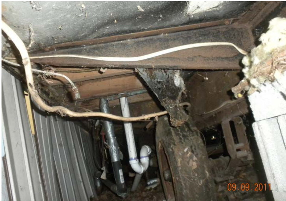
Crawl space under mobile home
