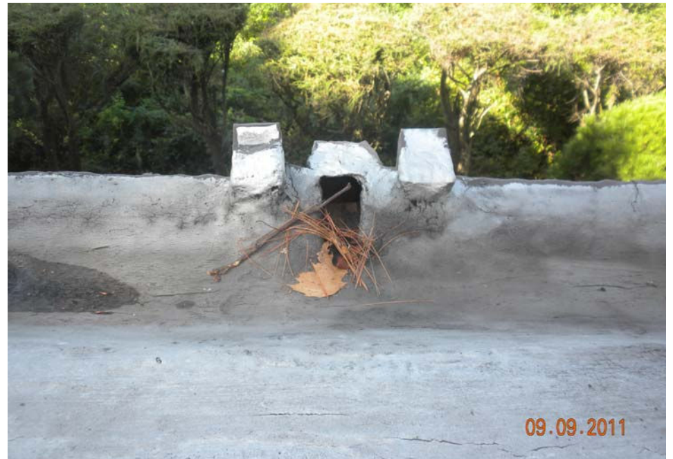
Roof Drain at main house
