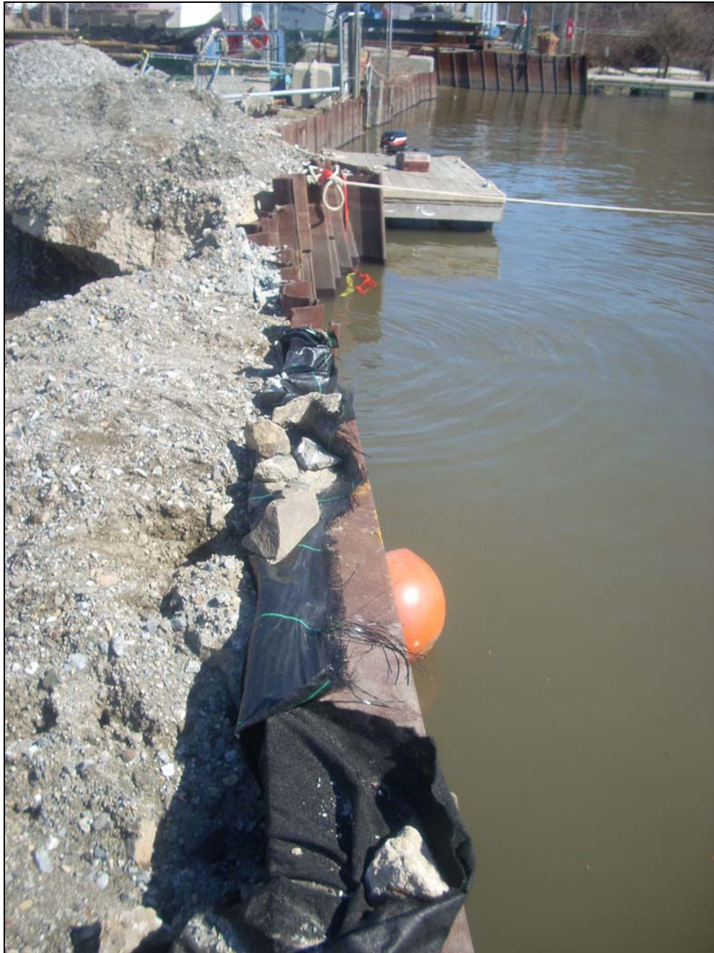
Photograph 6: Shoreline Segment D - South In-Building Area. View looking northeast. March 8, 2011.
