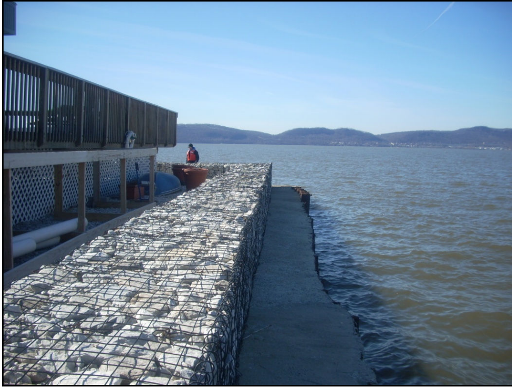
Photograph 3: Shoreline Segment A - I orth Building Area. View looking south. March 8, 2011.
