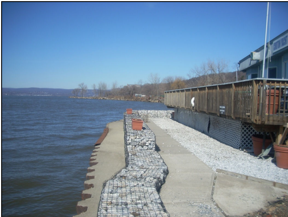
Photograph 4: Shoreline Segment B - Southwest Building Area. View looking west. March 8, 2011.
