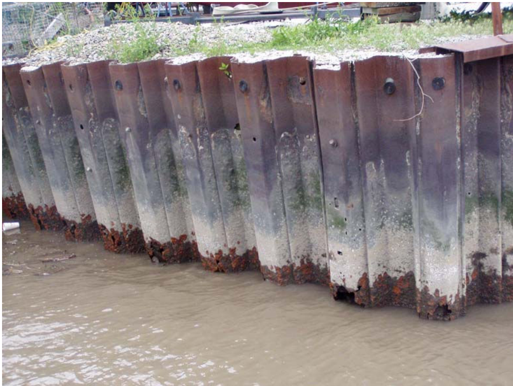
Photograph 7: Typical deteriorated condition of bulkhead. March 8, 2011.
