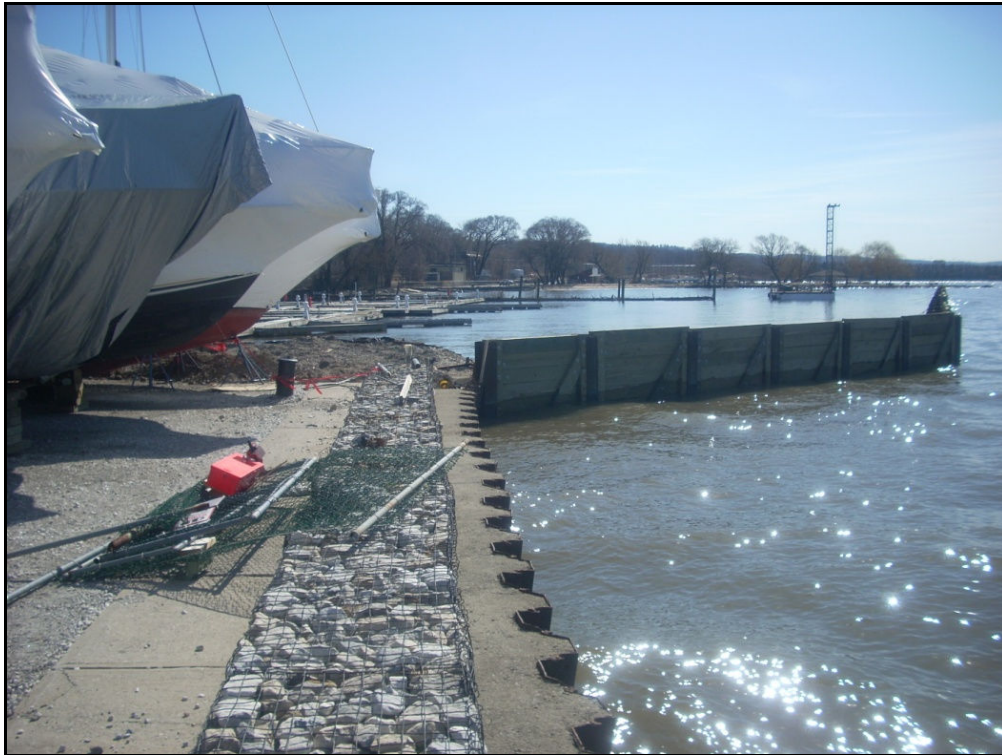
Photograph 5: Shoreline Segment C - Southwest In-Building Area. View looking east. Note timber wave screen and marina docks in background. March 8, 2011.
