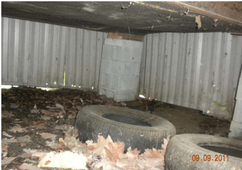
Crawl Space under Mobile Home
