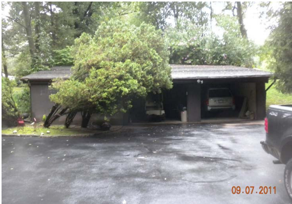
Two car garage with storage area
