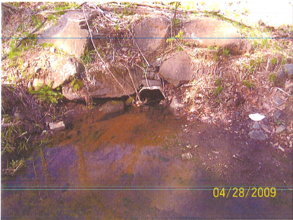
Existing 15"Ø Outlet Pipe
