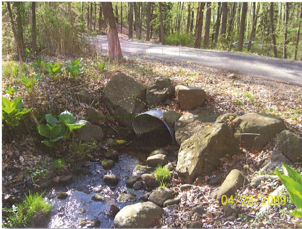
22" x 34" Elliptical Pipe Under Park Trail
