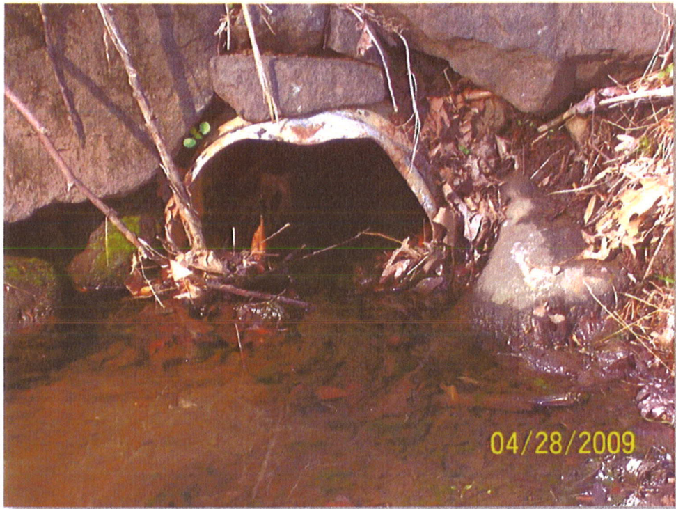
Existing 15"Ø Outlet Pipe
