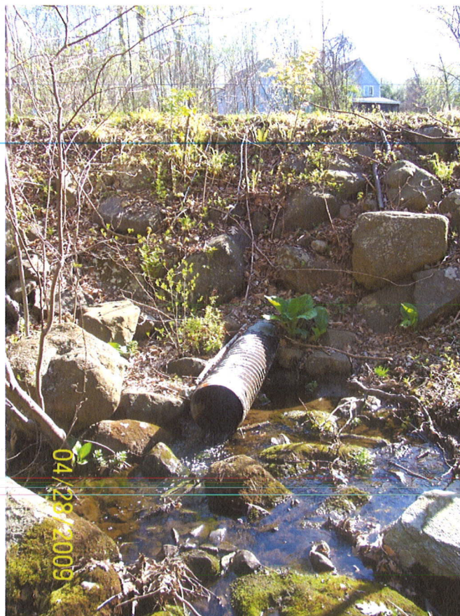
Downstream Side of 15"Ø Outfall Pipe
