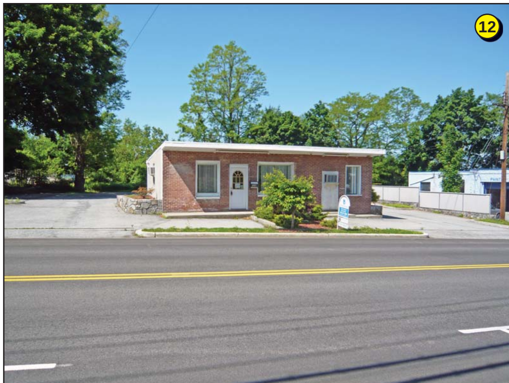
View southwest toward now-vacant one-story structure and parking areas on South Riverside Avenue.
