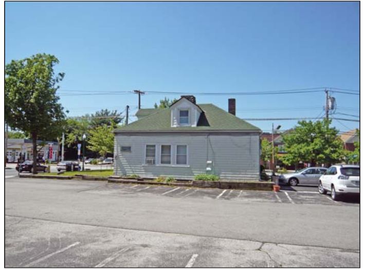
Rear of 73 Benedict Boulevard (view from parking lot).
