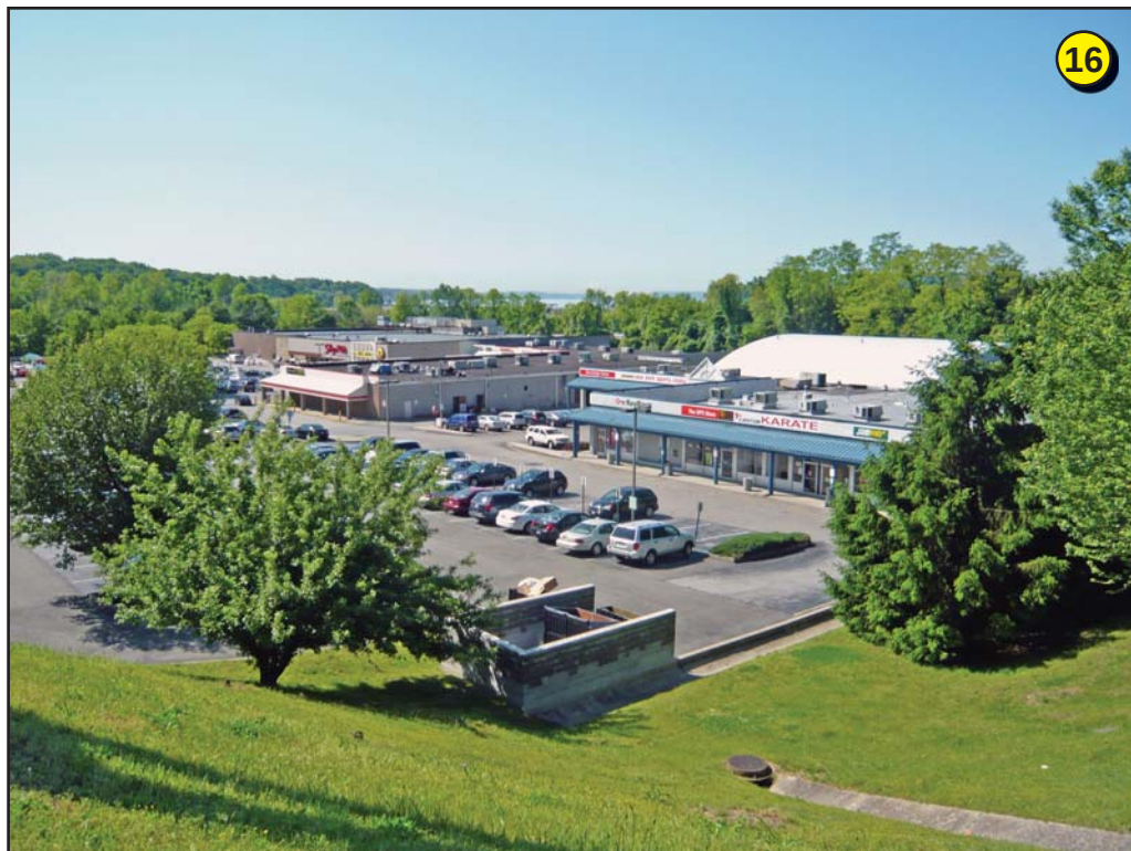
Outside H/SRG District; view south from South Riverside Avenue (south of its intersection with Croton Point Avenue). View of Hudson River in distance, beyond retail buildings.
