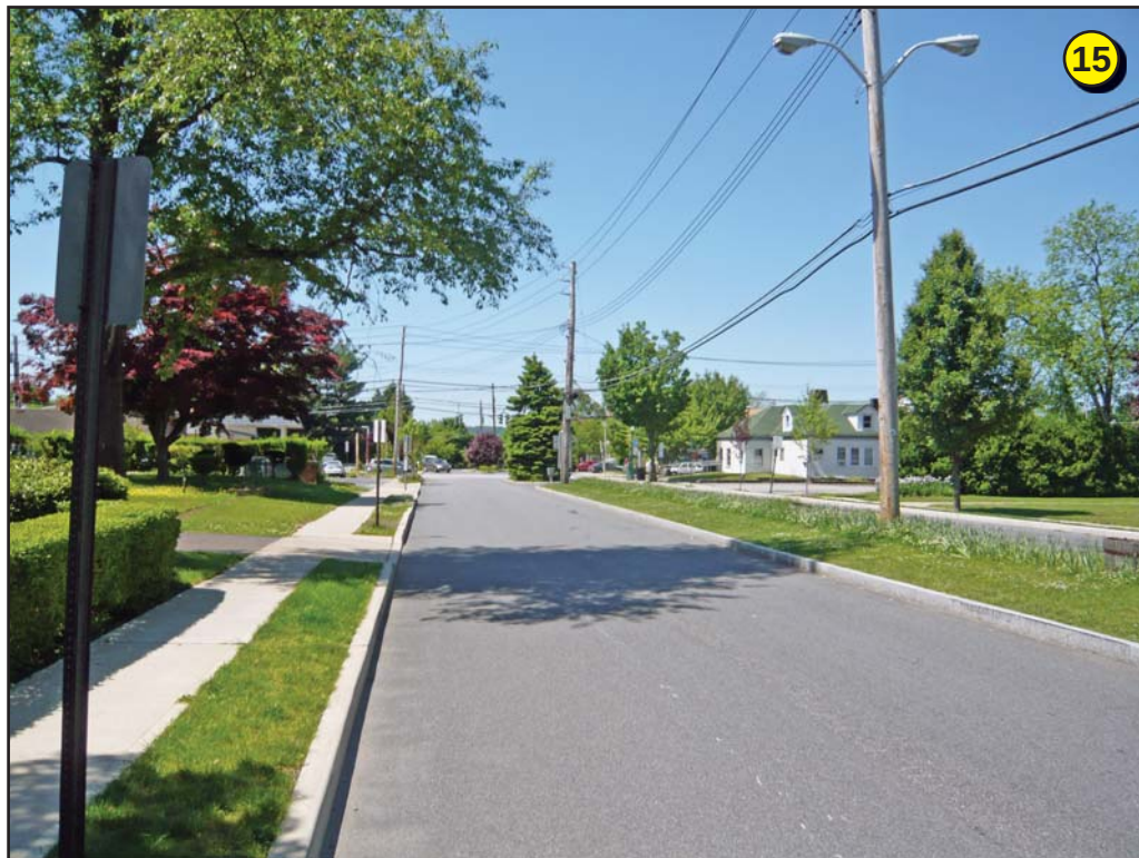
Outside H/SRG District; view southwest toward the gateway district from the intersection of Benedict Boulevard and Young Avenue.
