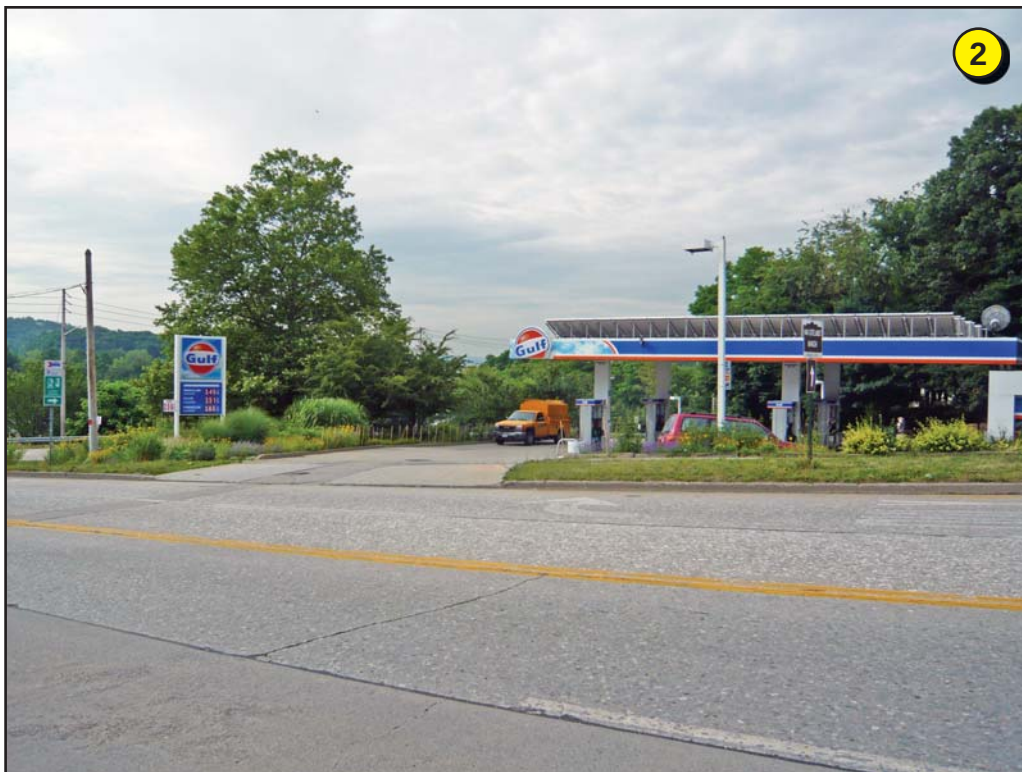
View south across South Riverside Avenue toward Gulf gas station with canopy on corner of Croton Point Avenue.
