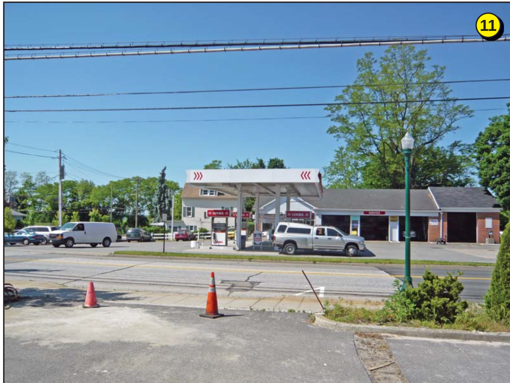
View southwest toward Luk Oil gas station on South Riverside Avenue.
