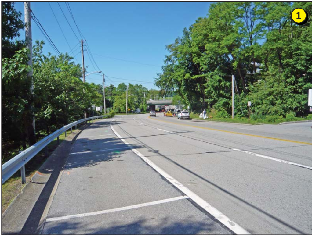
View of Croton Point Avenue (opposite Gulf gas station), looking southwest toward Route 9.
