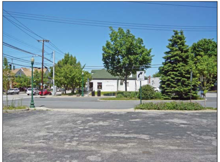
73 Benedict Boulevard as viewed from vacant parcel on southeast side of Benedict Boulevard.
