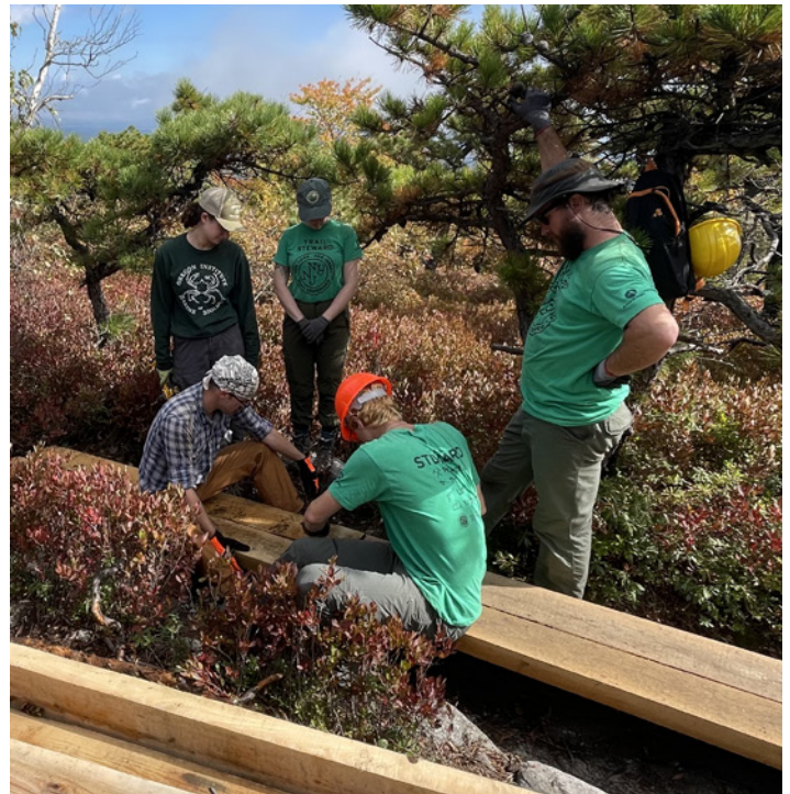
Building bog bridges at Sam's Point, photo by Myra Romano
