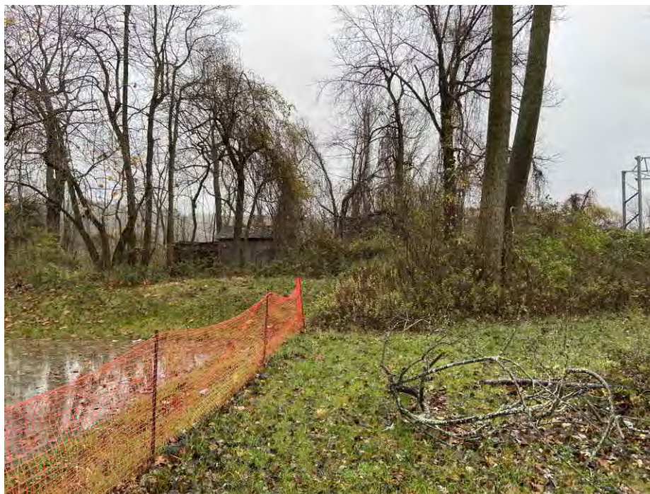
Photo 4: Stormwater detention basin, facing southeast.
