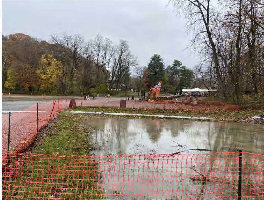
Photo 3: Stormwater detention basin, facing northeast
