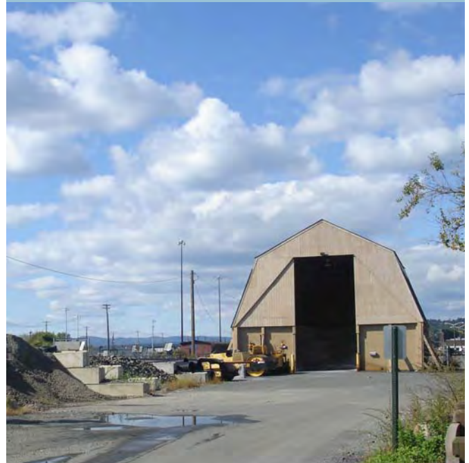
Figure 2-27. Municipal Garage, Croton
