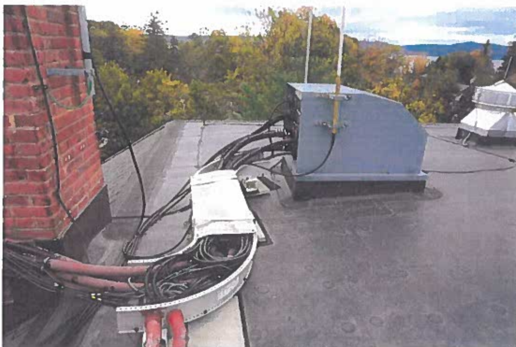
Photo 4: T-Mobile Typical Cable Routing
