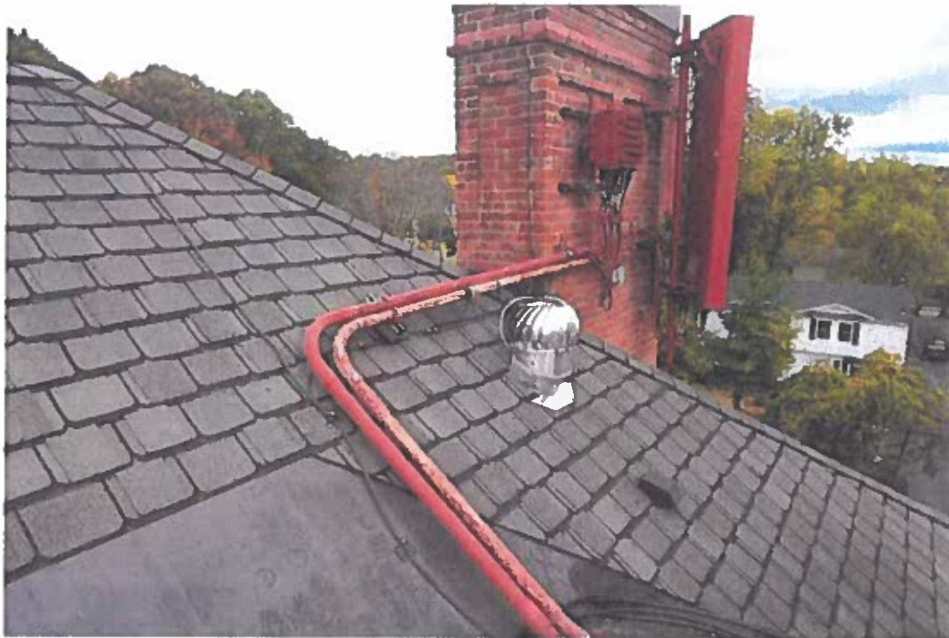
Photo 5: T-Mobile Typical Cable Routing
