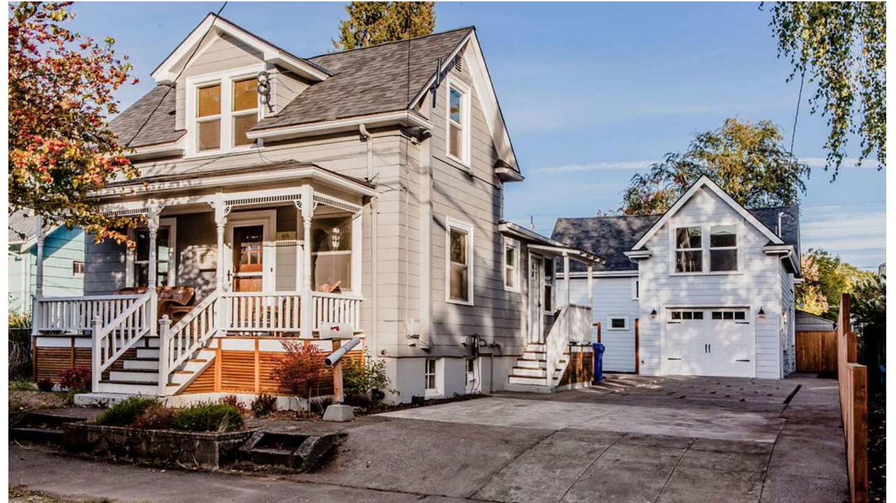
Converted Garage in Delaware
