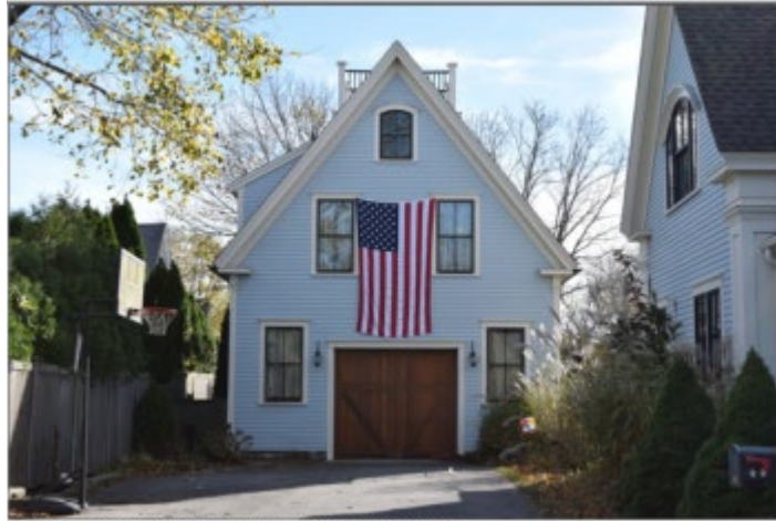
Photo 3. Barn at 275 Old Main Street, looking southwest.
