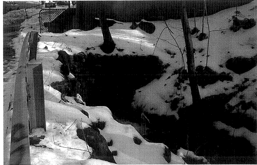
Outlet at Lot 23 on Brook Street
