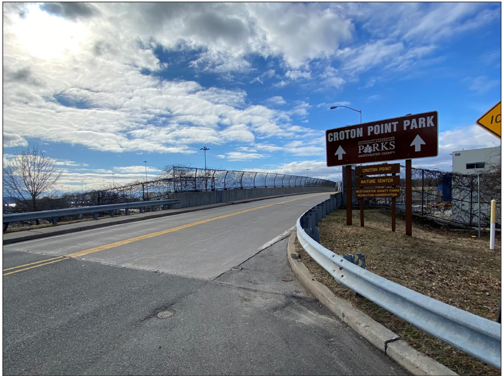
View west along Croton Point Avenue 2
