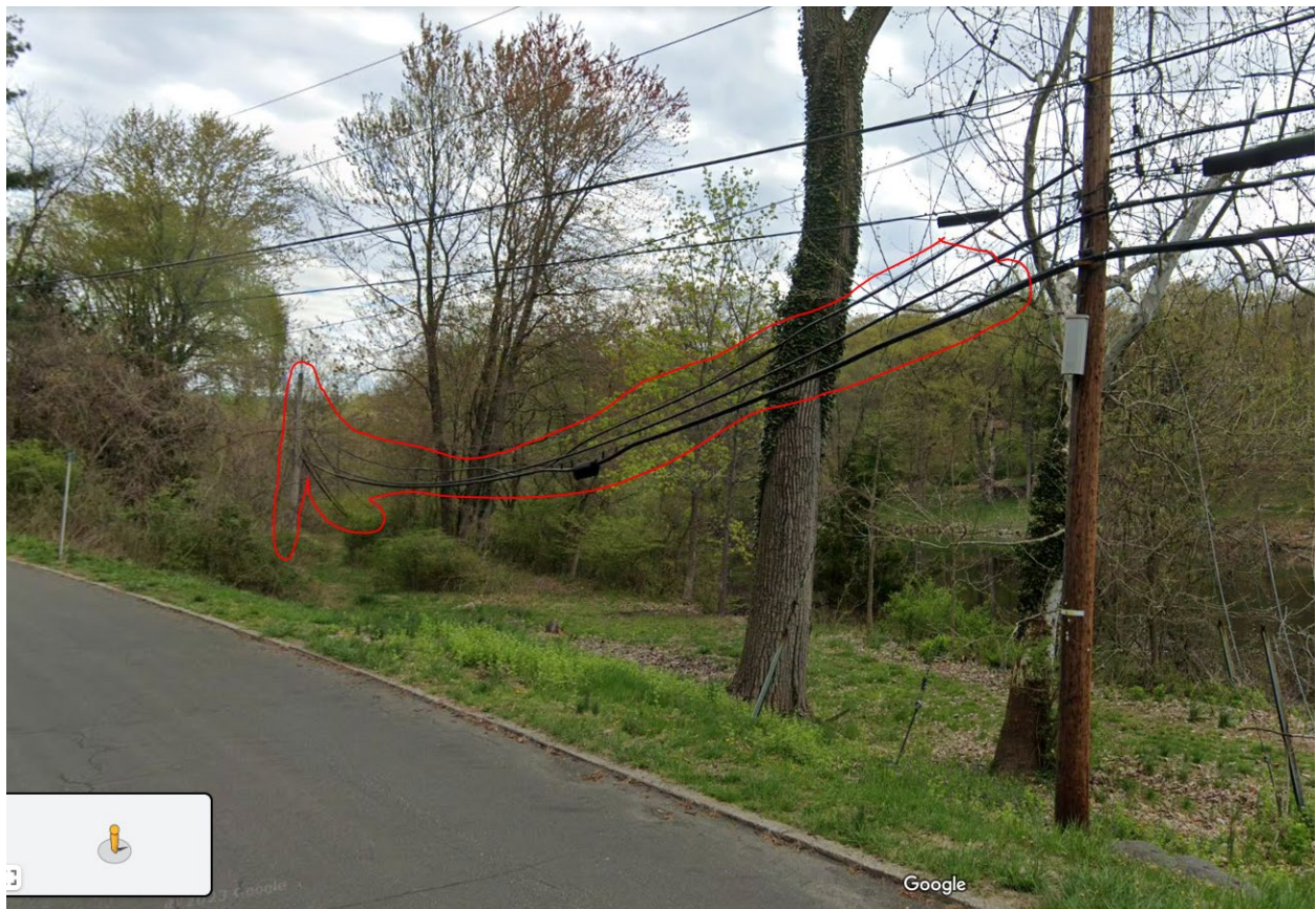
Image showing part of old telecommunication cables and poles to be removed (items circled in red)
