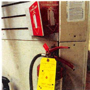
M&J Auto Fire Inspection Photo
