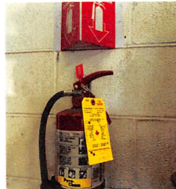
M&J Auto Fire Inspection Photo
