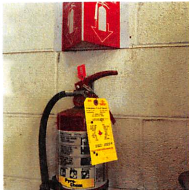
M&J Auto Fire Inspection Photo
