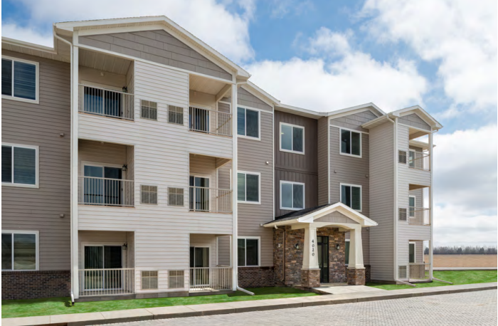
Regency Apartment Homes (144 units) Williston, ND
