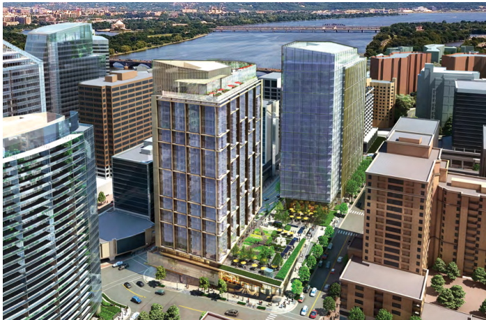
1400 Key and 1401 Wilson Redevelopment (800 Units) Arlington, VA
