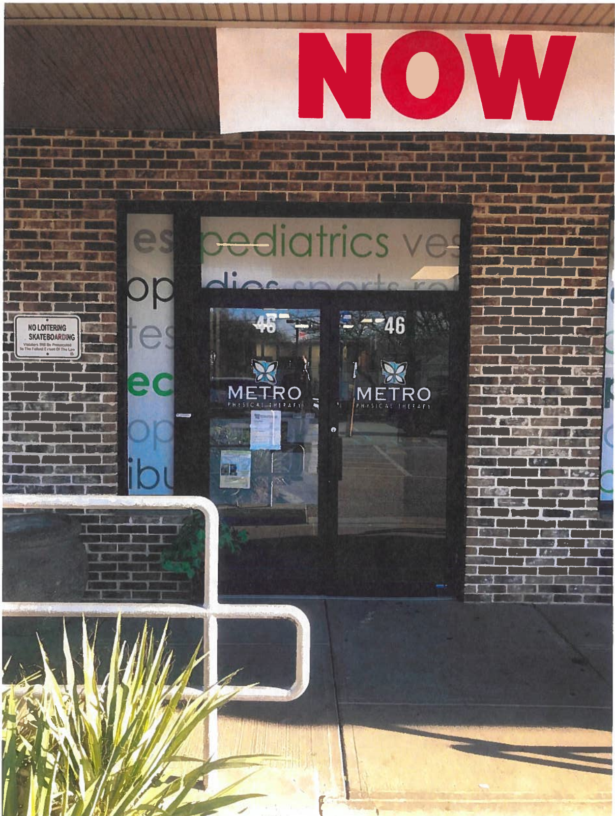
Sign covers 100% of windows.
