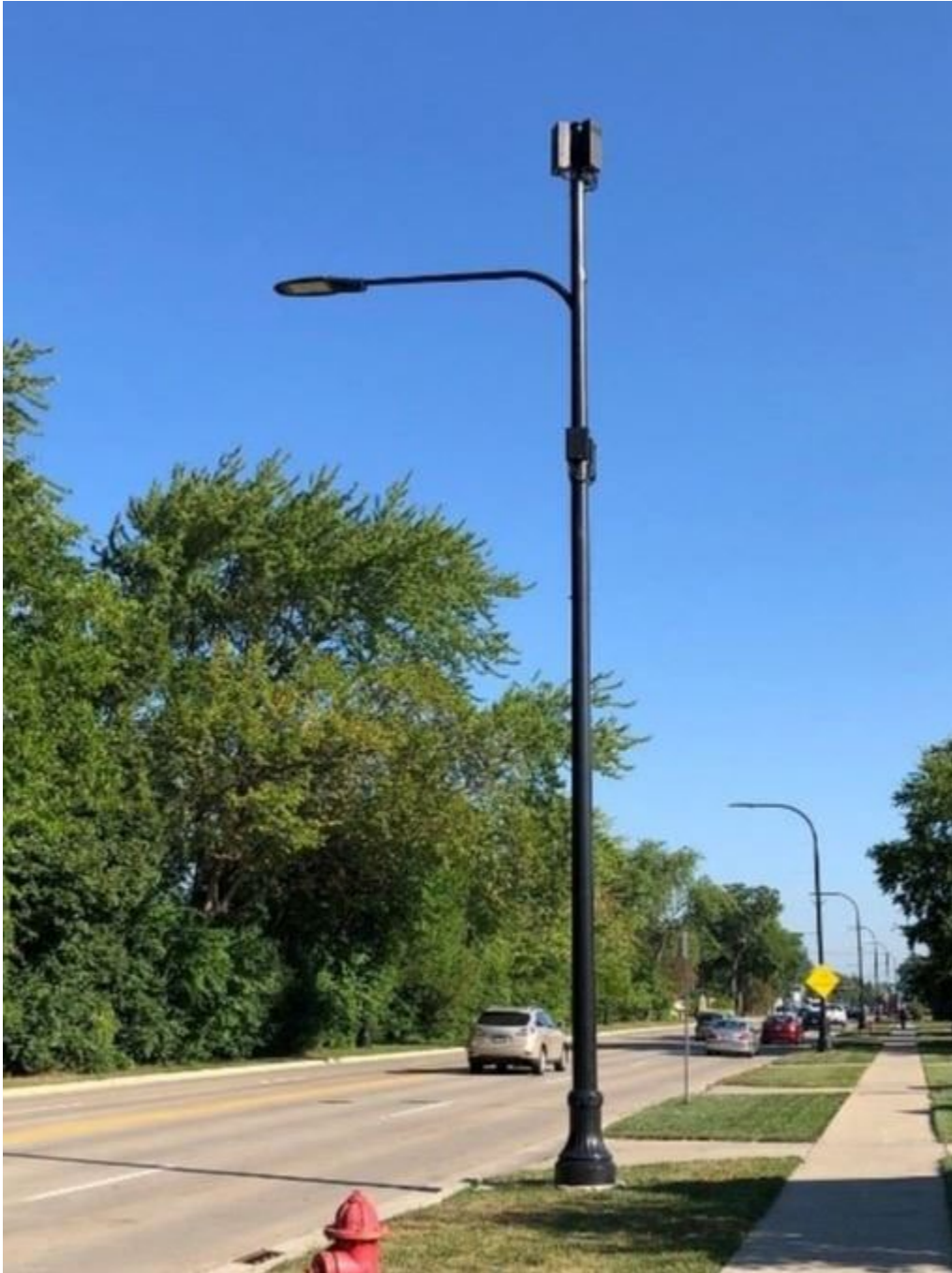
Small Wireless Facility: Black “integrated” pole with streetlight design.
