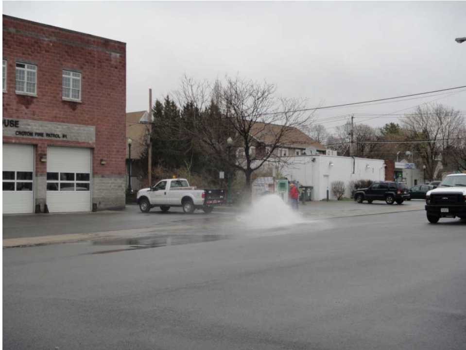
Hydrant A (Benedict Blvd.): Flow rate was 1120 GPM.
