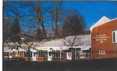
Croton Professional Building along Riverside Avenue
