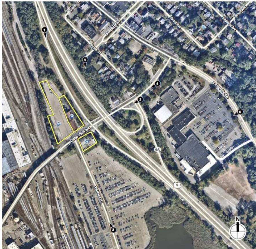
VIEW POINT 3 PRESENTS THE WESTERLY VIEW OF PARCELS 48-50 FROM THE INTERSECTION OF CROTON POINT AVENUE AND THE OFF-RAMP EXITING NORTHBOUND ROUTE 9.
