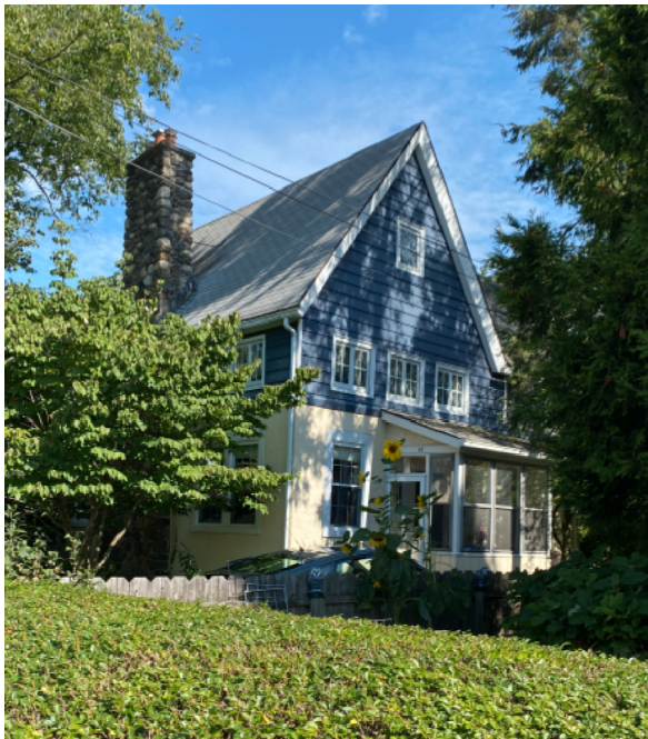
HOUSE FROM SOUTH WEST
