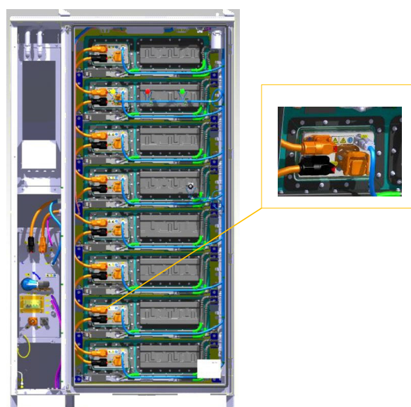
Figure 12. Installation of MSD
