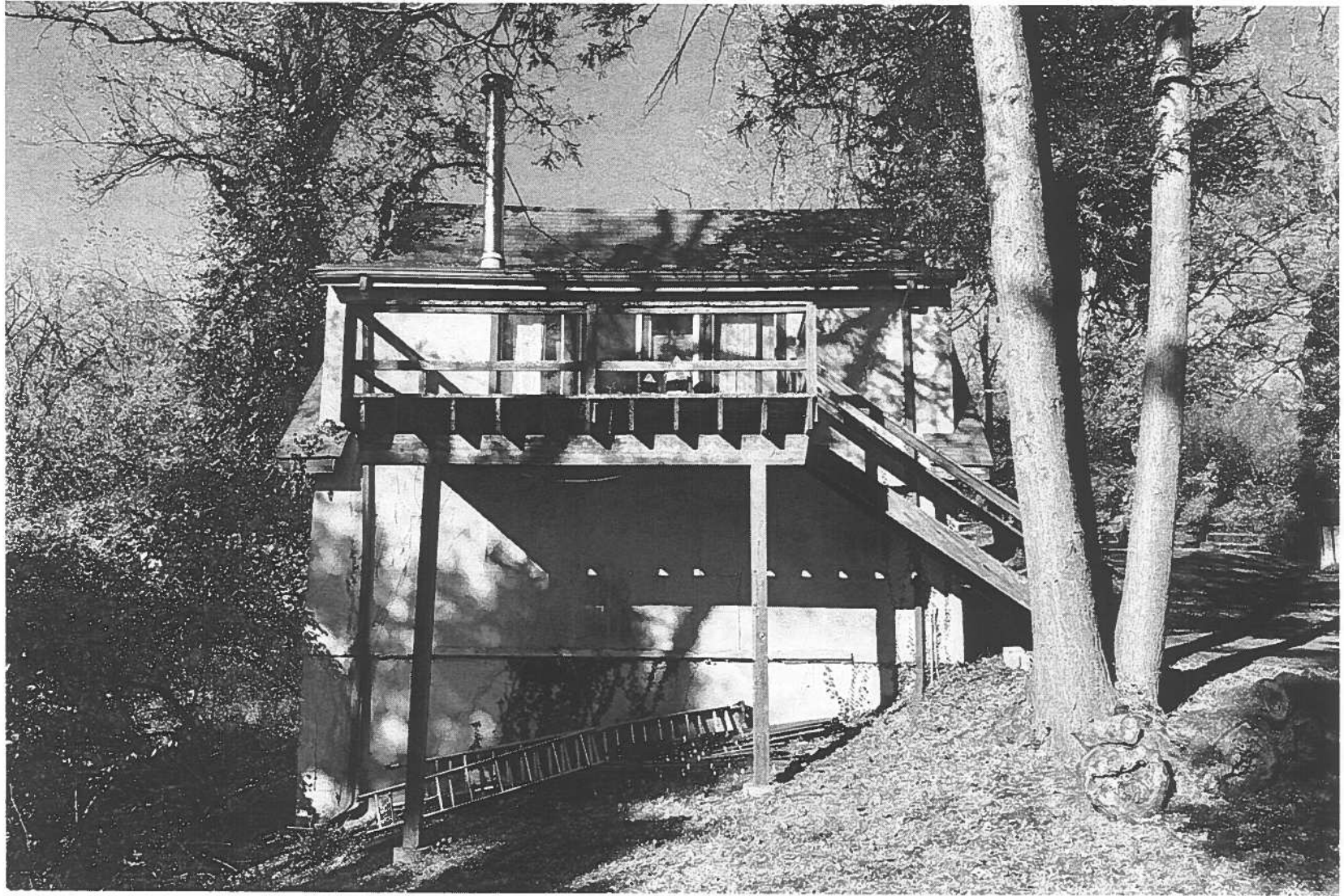
Garage Left side. View from the Main House.
