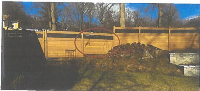
Removed horizontal slats on steeper elevations to minimize height gain.
