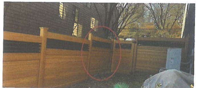
Removed horizontal slats on steeper elevations to minimize height gain.
