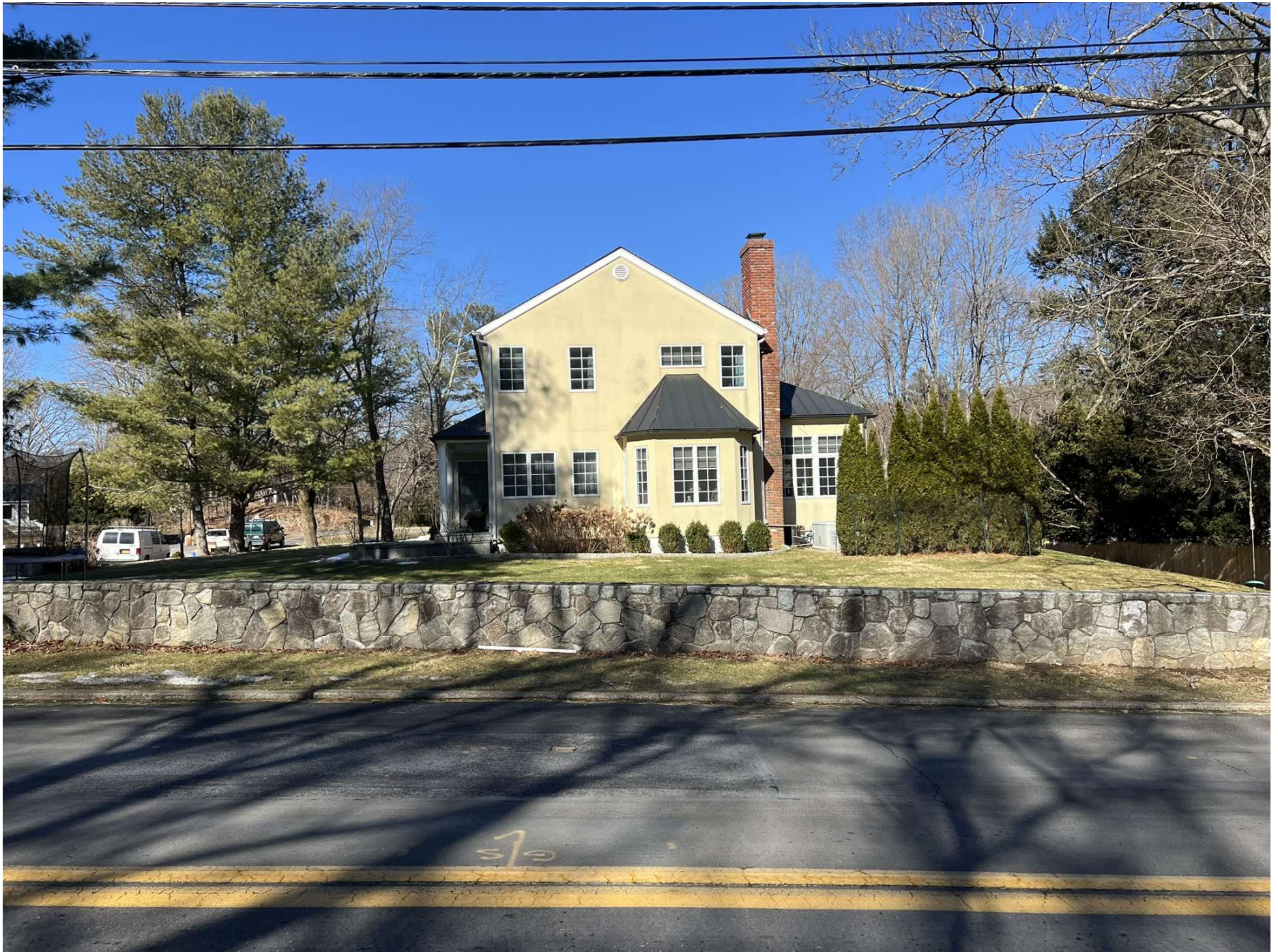
2 Kuney Street (neighbor to left)
