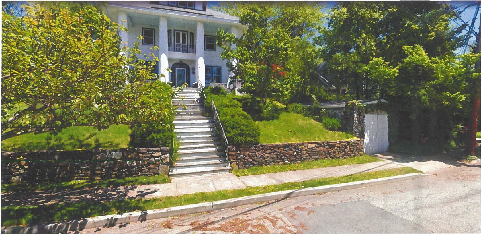
16 LEXINGTON DRIVE - STREET VIEW EXISTING
