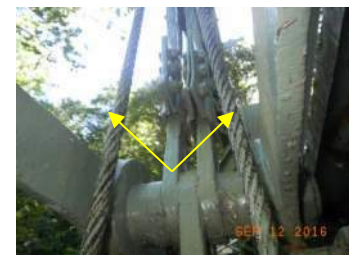
Existing truss members retrofit with steel cables
