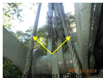
Existing truss members retrofit with steel cables
