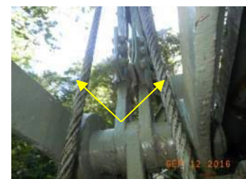
Existing truss members retrofit with steel cables
