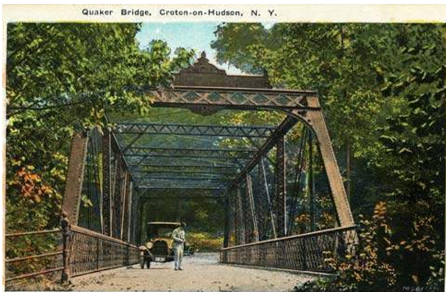
Figure 5. Postcard view, c. 1930. This view shows the original railings in place, and the original location of the date plaque, which was attached to the bottom of the portal lintel.
