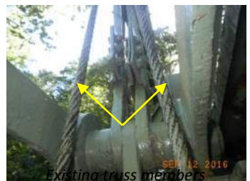
Existing truss members retrofit with steel cables
