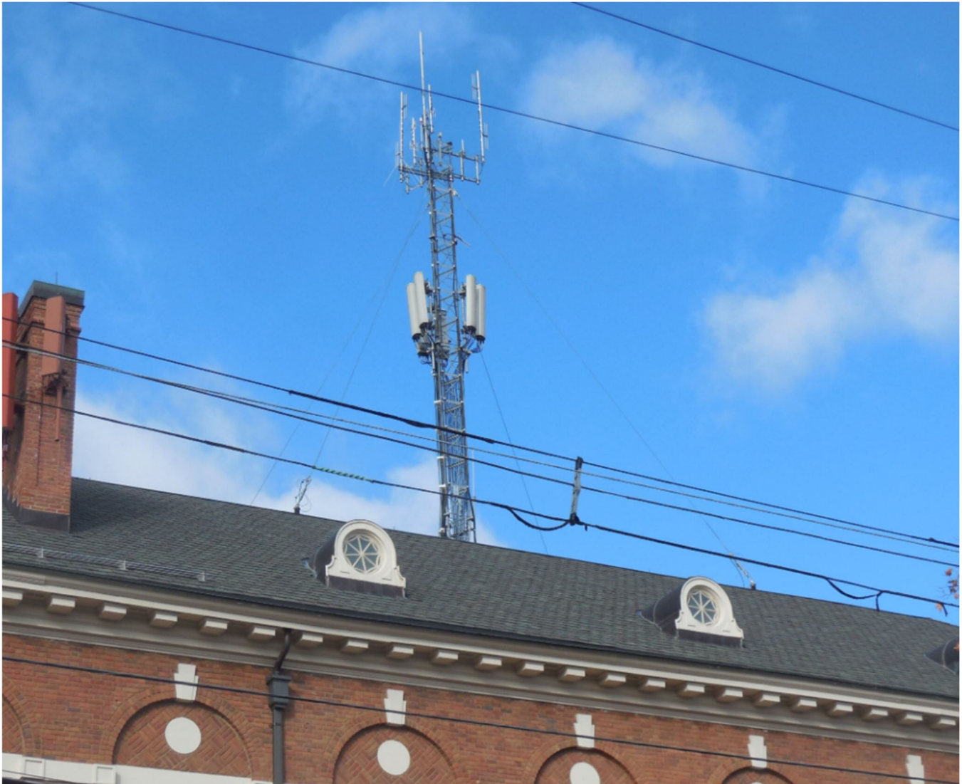
GUYED TOWER OVERALL VIEW
