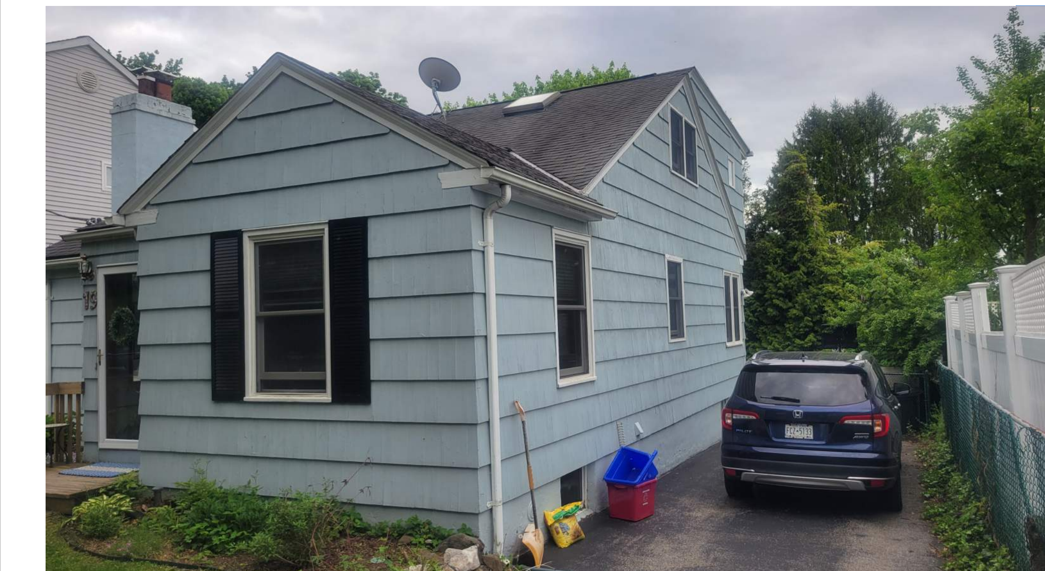
Side View - West
