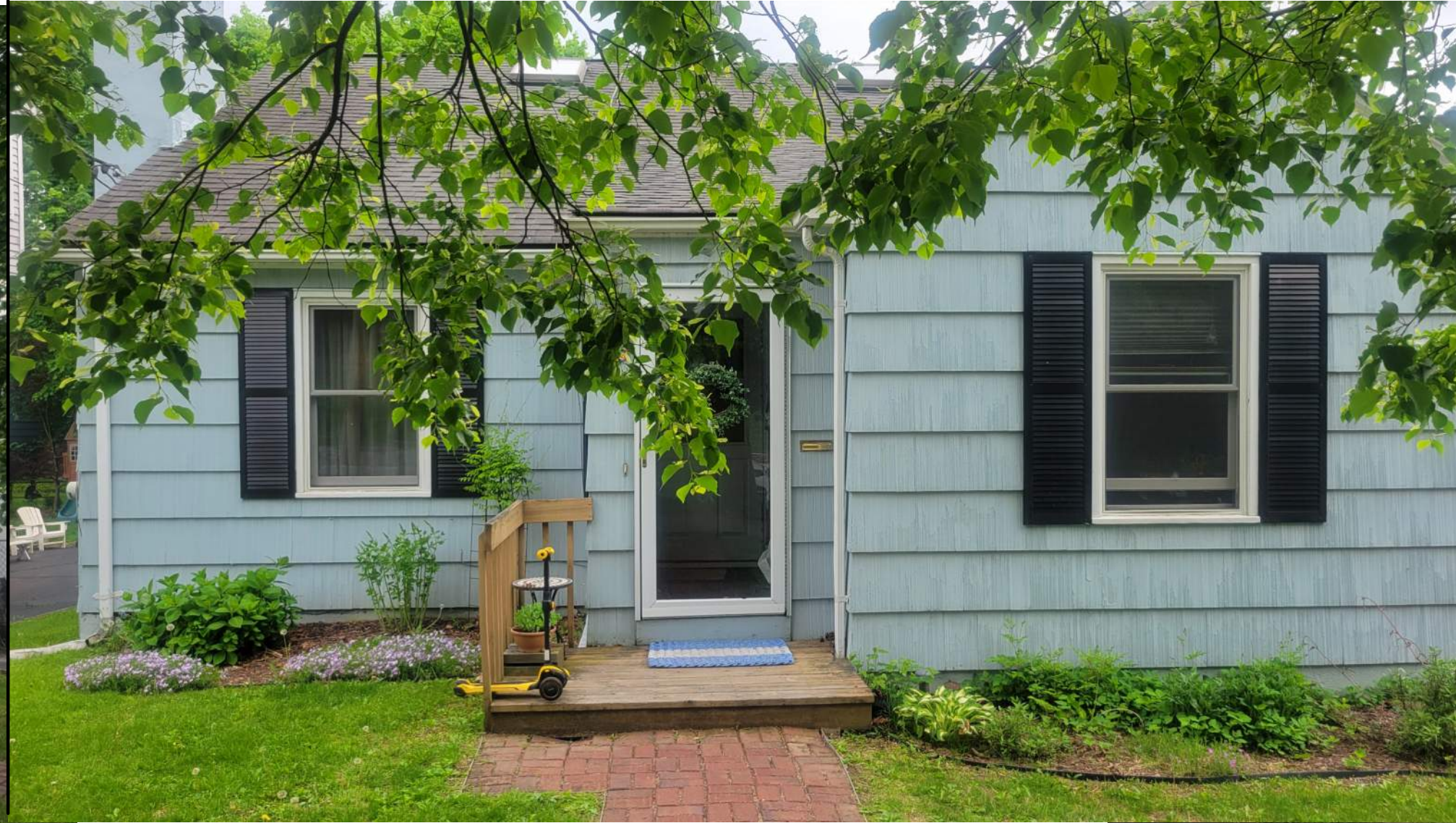
Front View - North
