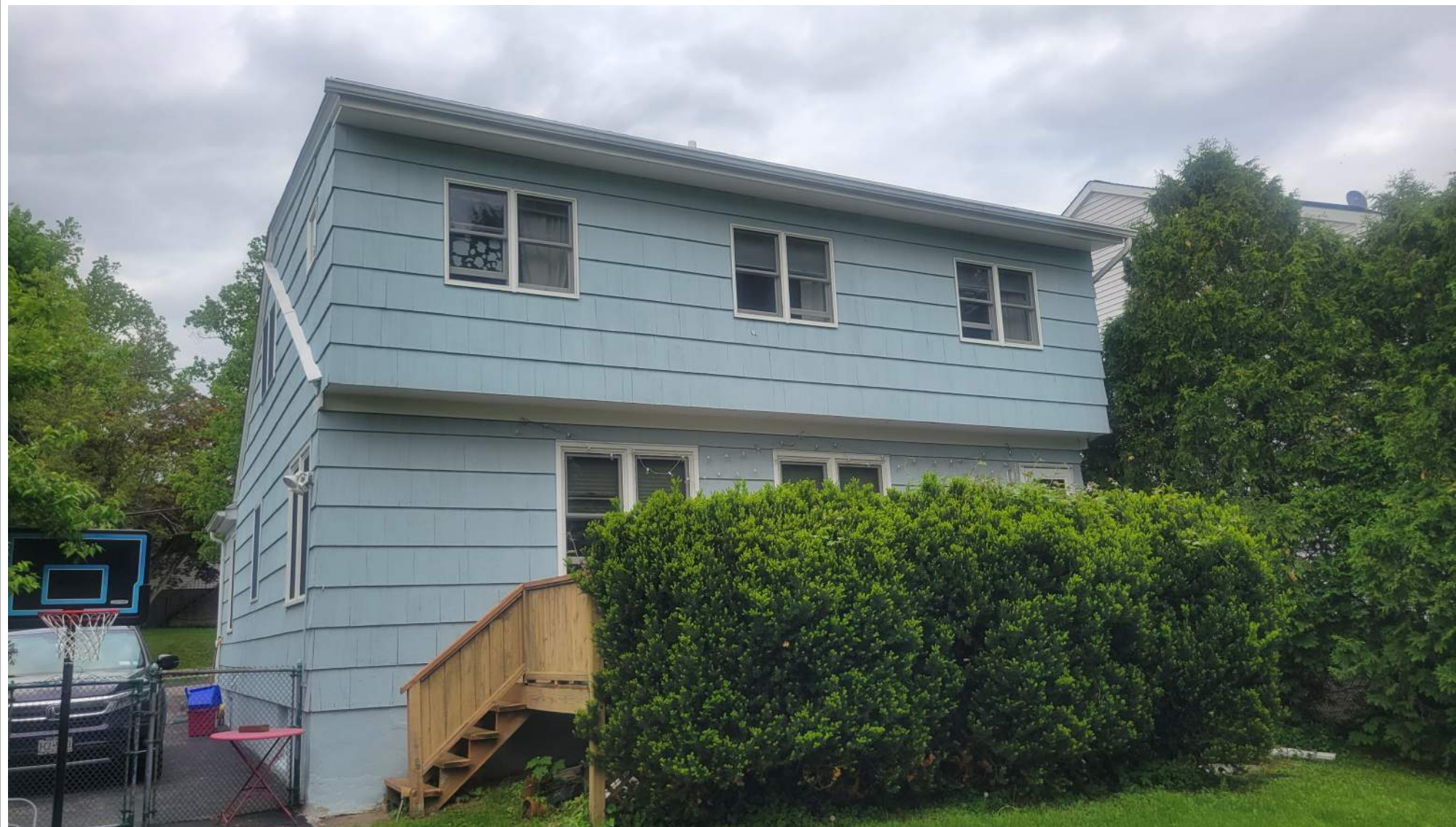
Rear View - South Side
