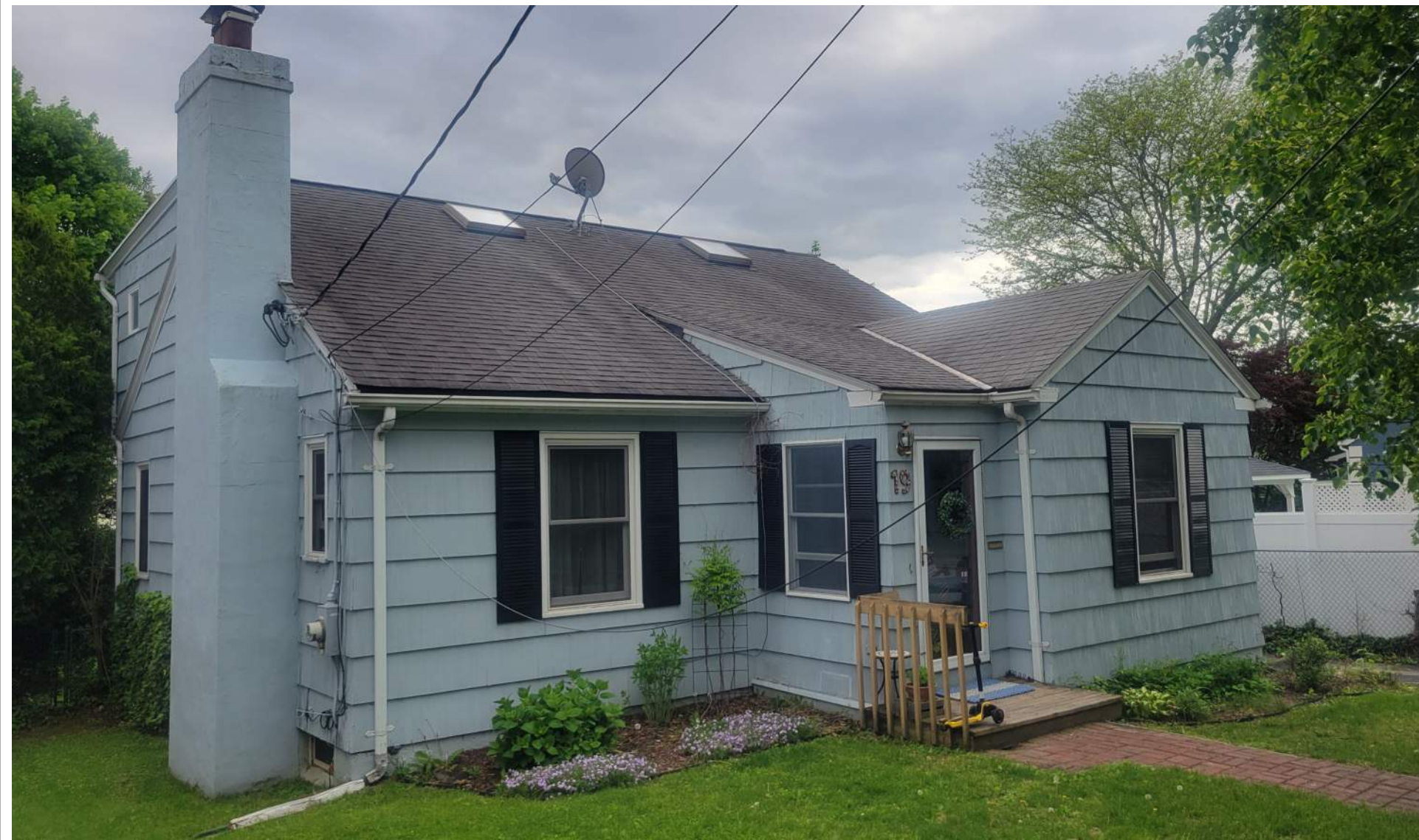
Front View - North
