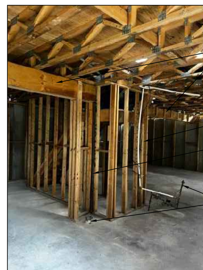
PHOTO OF REMAINING CONSTRUCTION AT FORMER MECHANICAL SPACE
