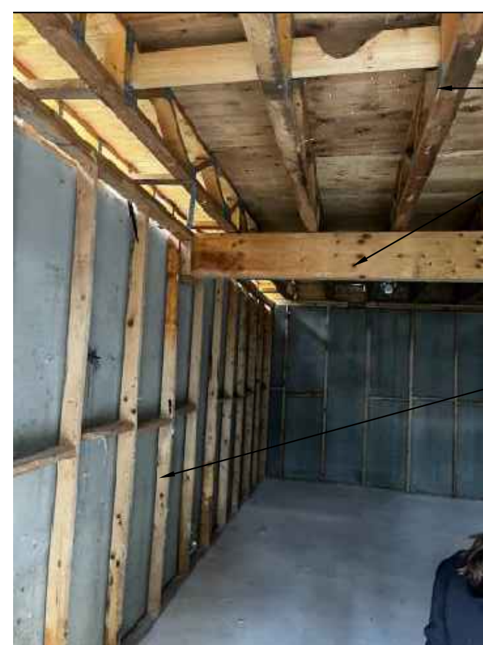
PHOTO OF REMAINING CONSTRUCTION ALONG FOUNDATION WALL, TYPICAL
