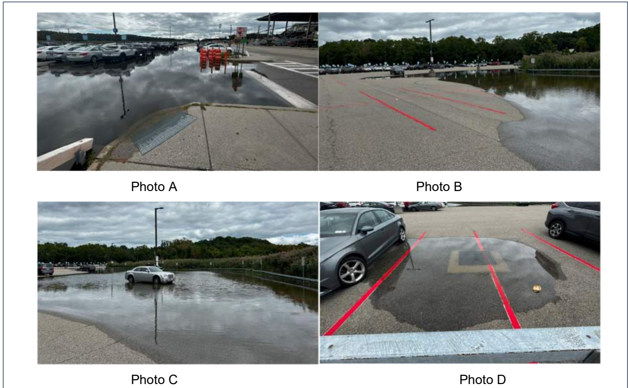
Figure 2. Photos taken during site visit on 9/20/2024 by AKRF.
