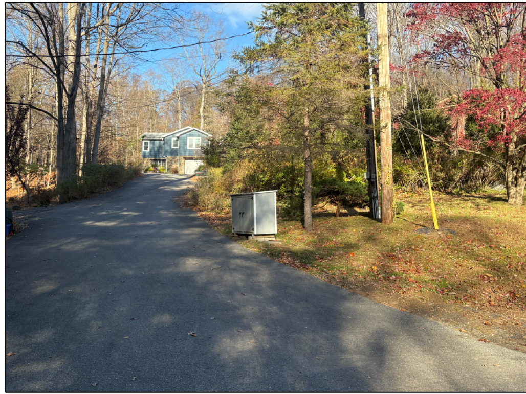
View Looking Northwest - 43 Riverview Trail N.T.S.
