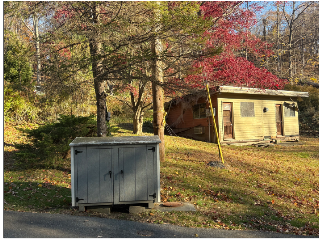
View Looking Northwest - 43 Riverview Trail N.T.S.
