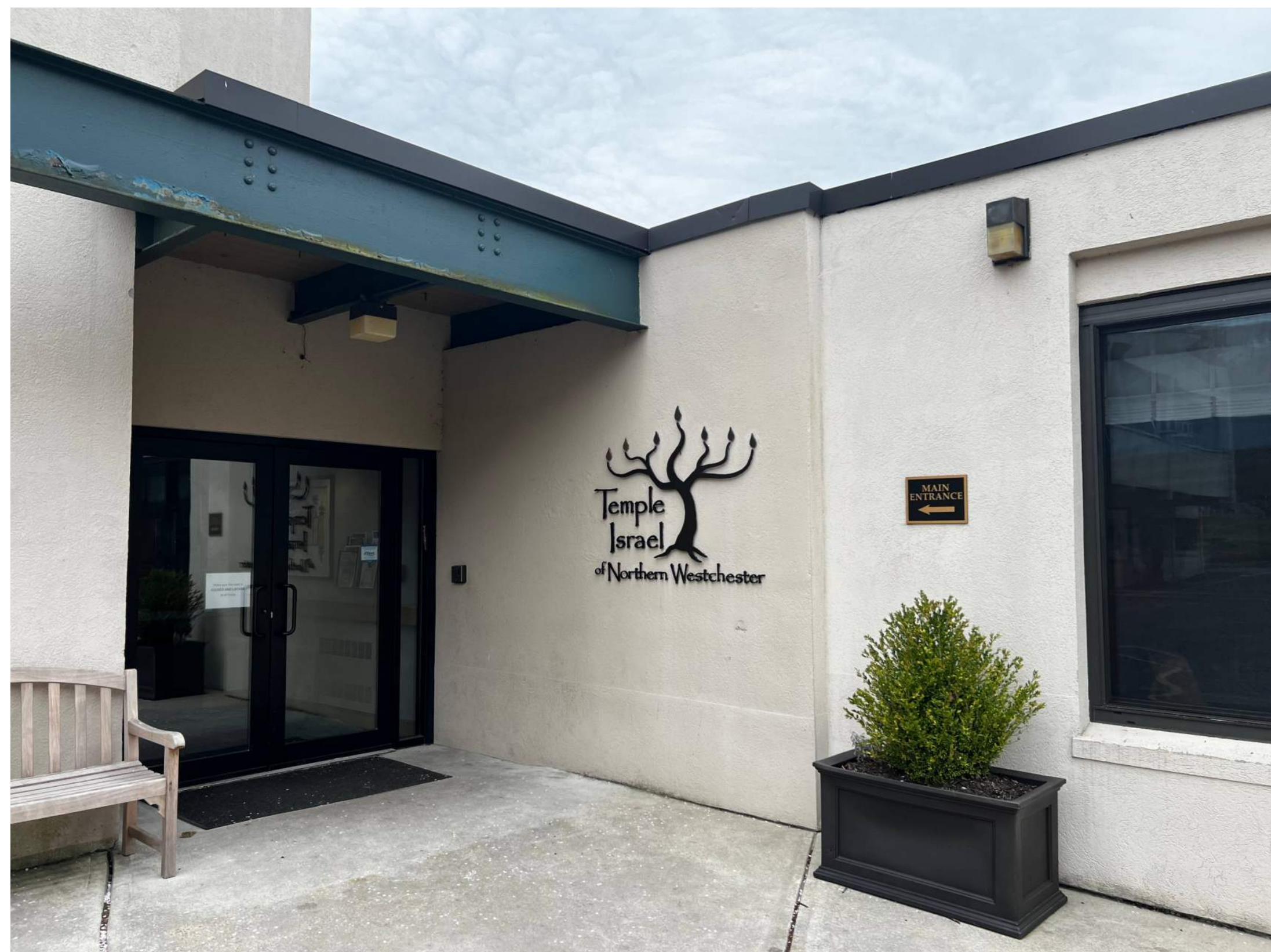
VIEW OF EXISTING NORTH ENTRANCE (CLOSE UP)
