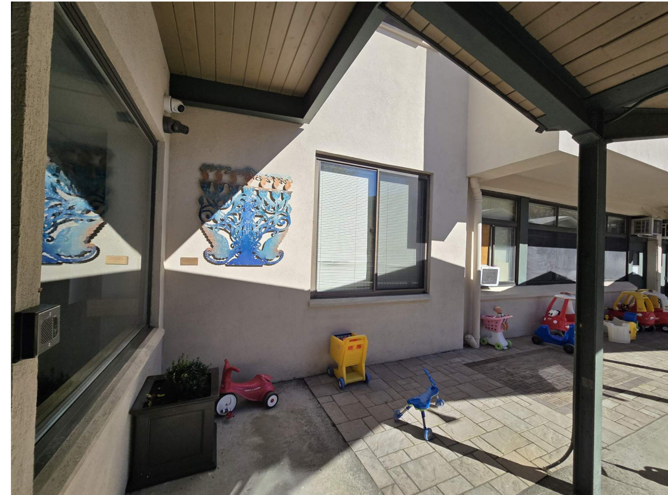
VIEW OF EXISTING SOUTH ENTRANCE
