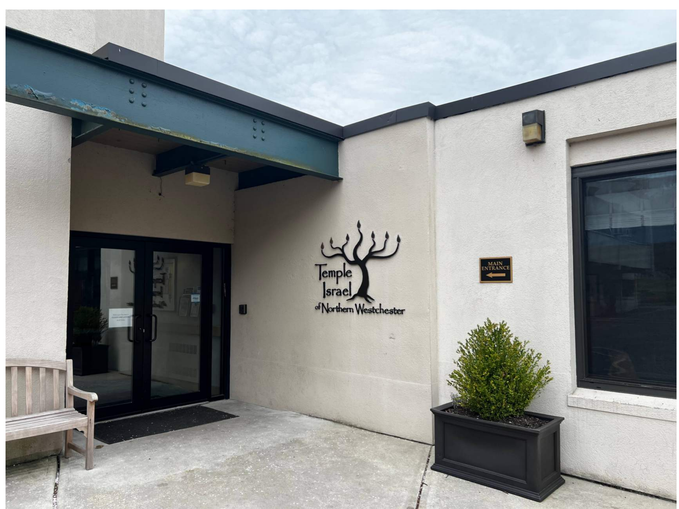
VIEW OF EXISTING NORTH ENTRANCE (CLOSE UP)
