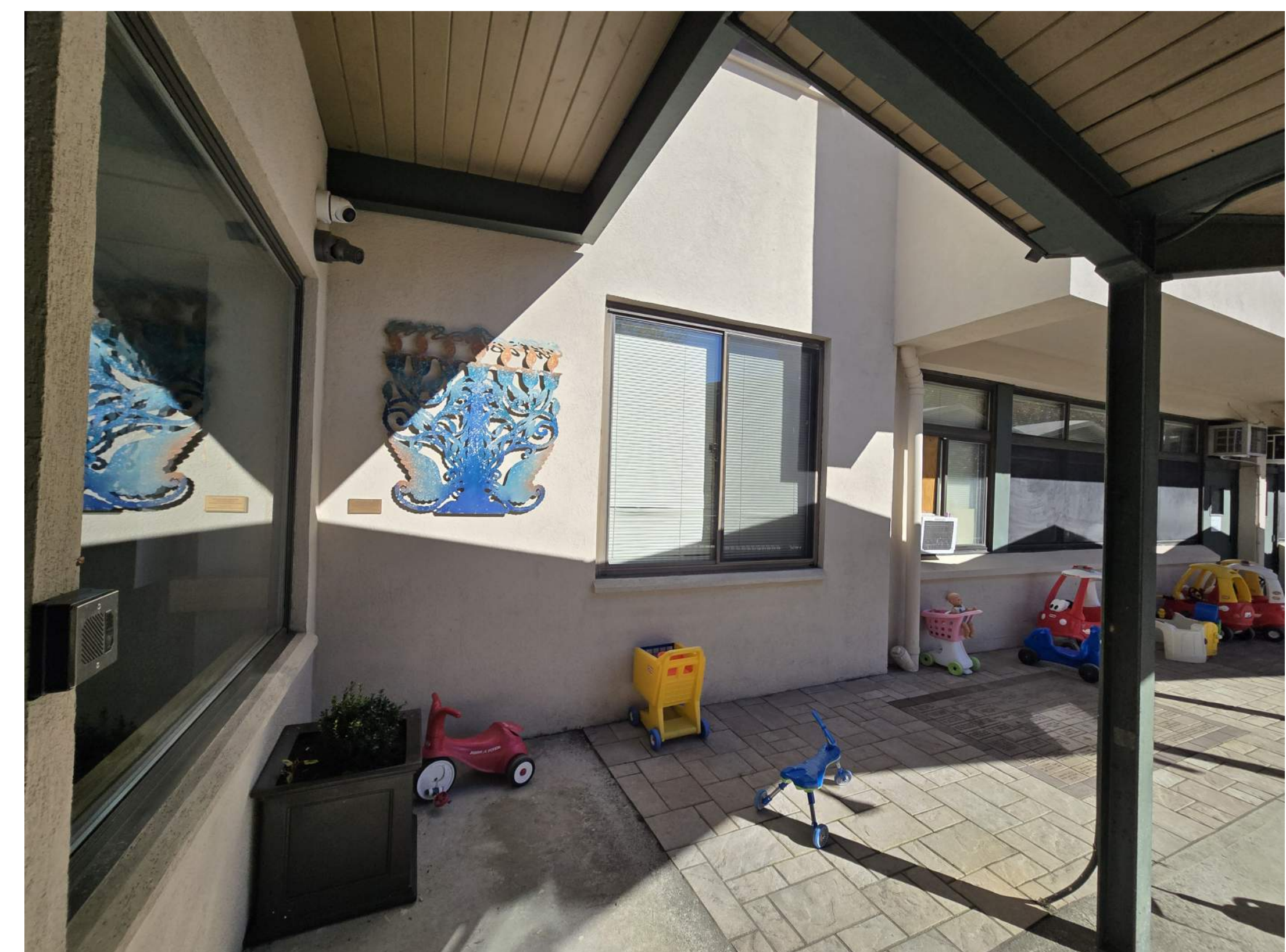
VIEW OF EXISTING SOUTH ENTRANCE
