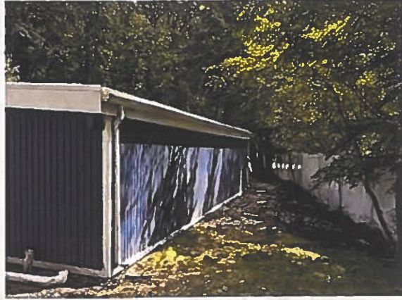
Garage Rear & Fence Line
