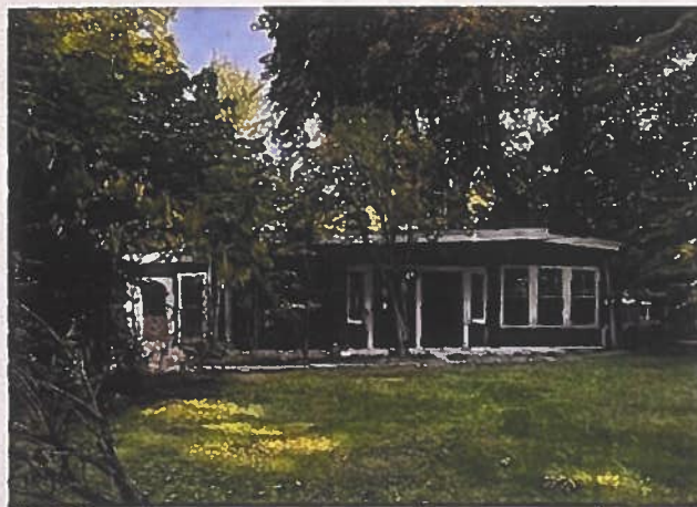
Front Yard View
