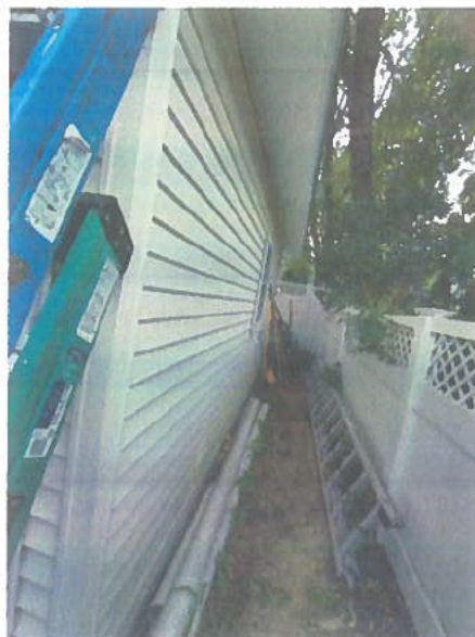
REAR AND SIDE OF EXISTING GARAGE
