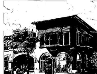
2. Precedent Example of building variety, color, mass, shape and material
