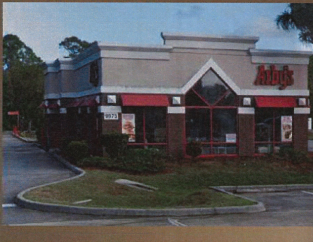
Existing Front Façade
