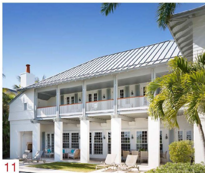
11 Standing seam metal roof, rhythm of balcony columns, building base
