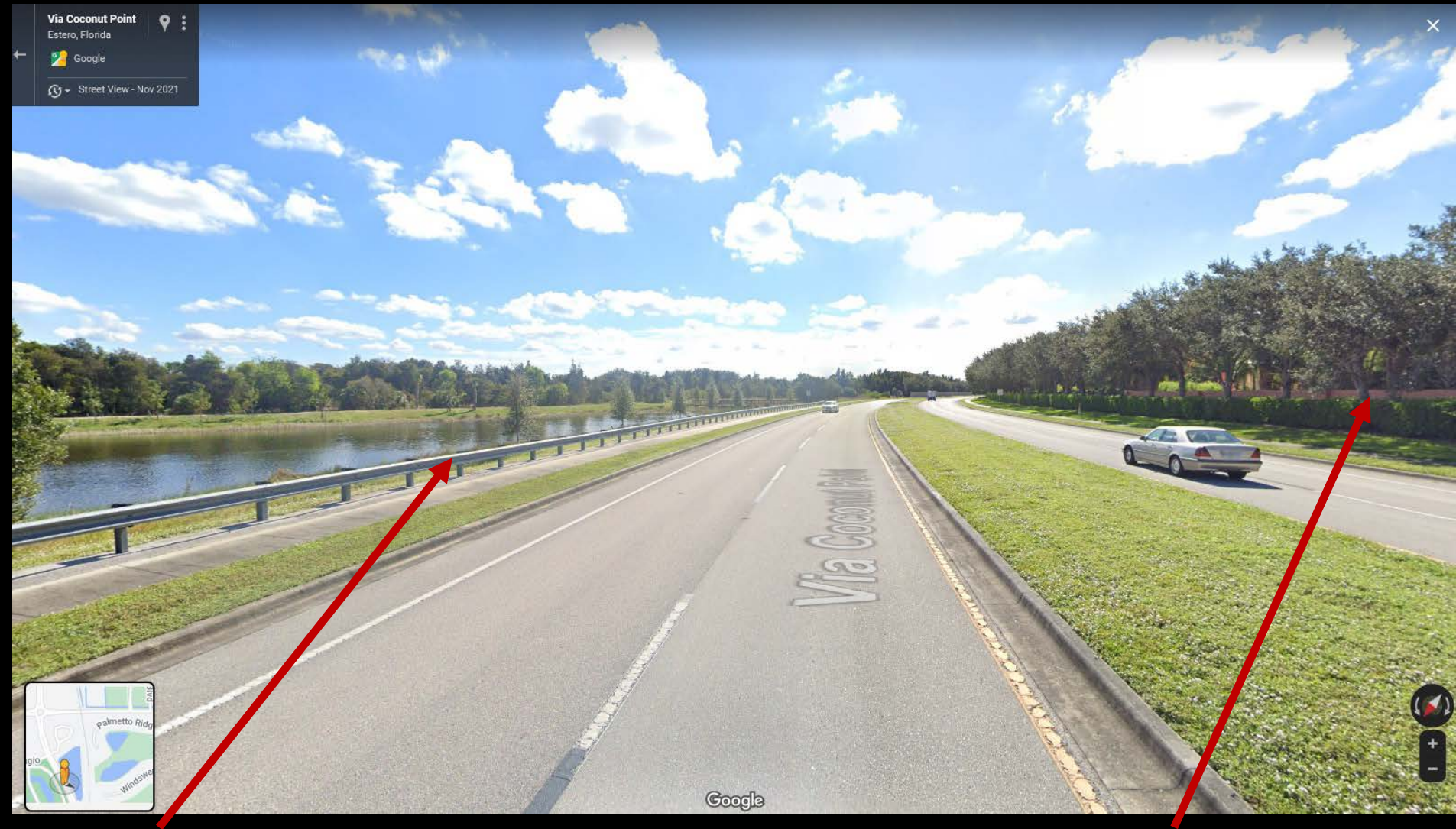
Guardrail along pond
