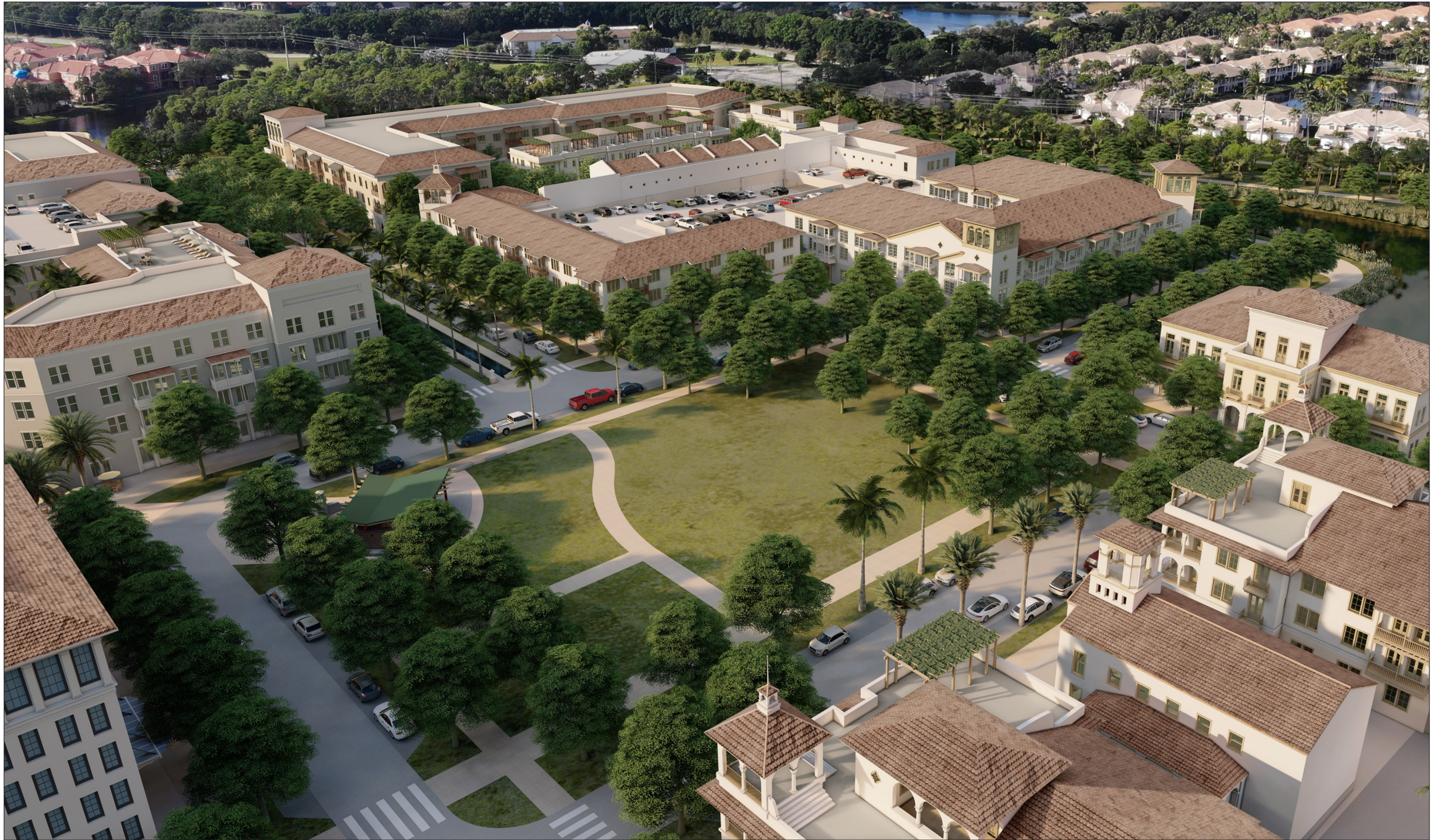
Central Green Aerial View: At the Civic Building site looking southwest
