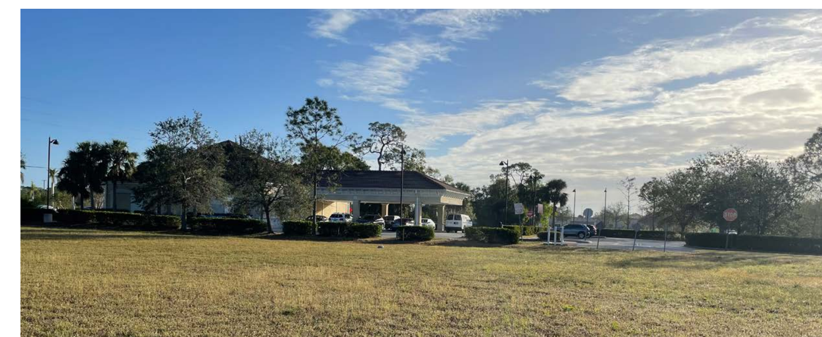
D. EXISTING EAST BUFFER
