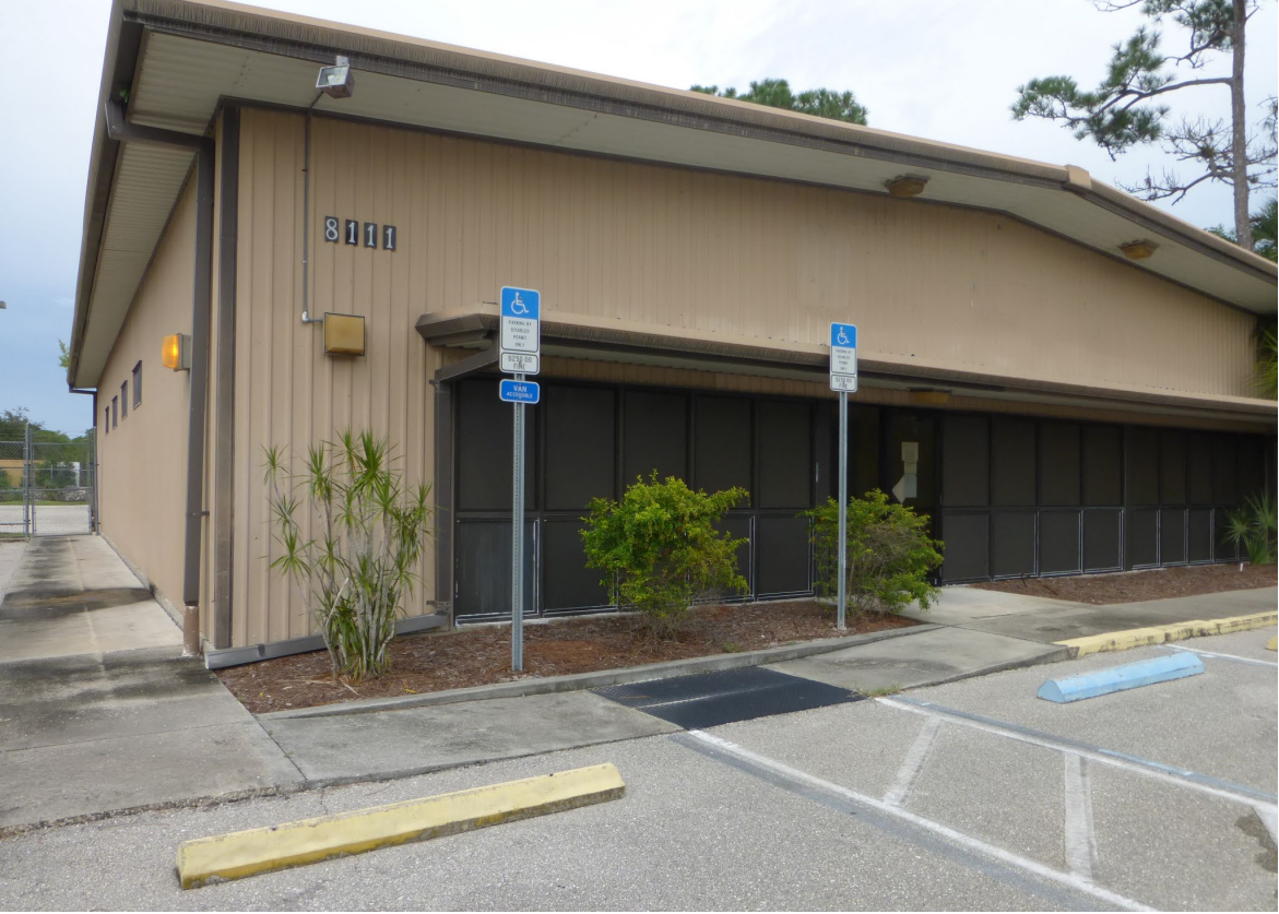
EXISTING BUILDING FRONT FACADE
