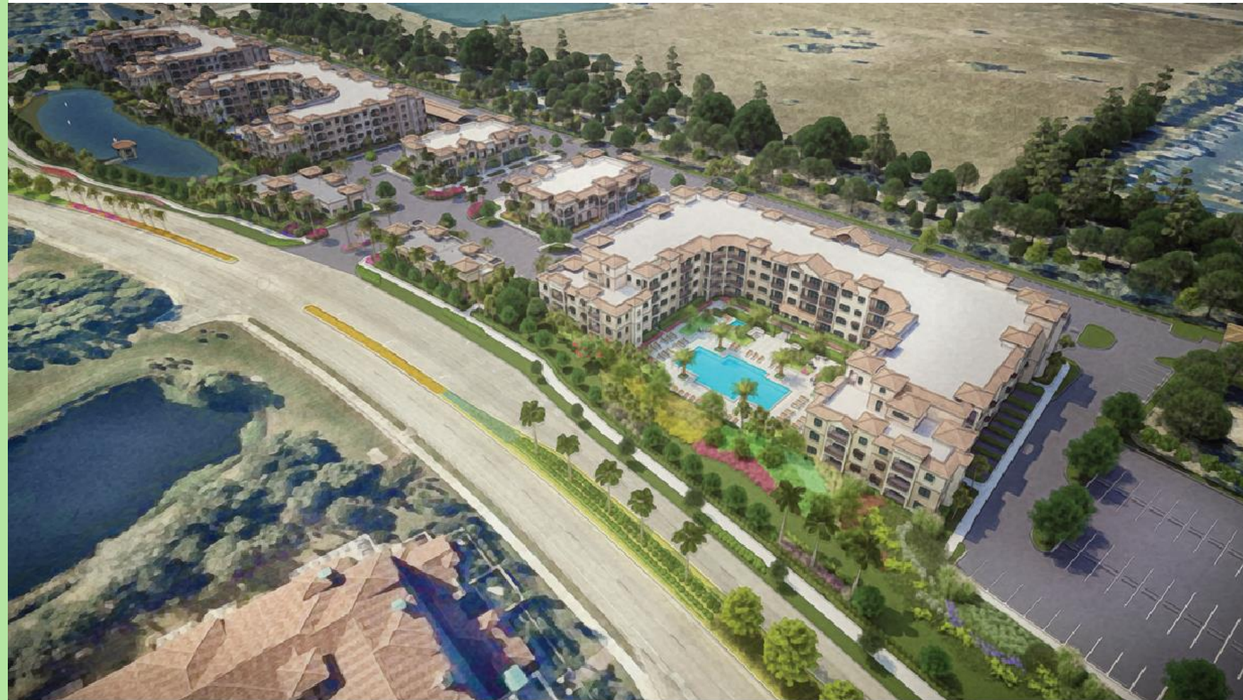
OVERALL AERIAL VIEW FROM NORTHEAST
