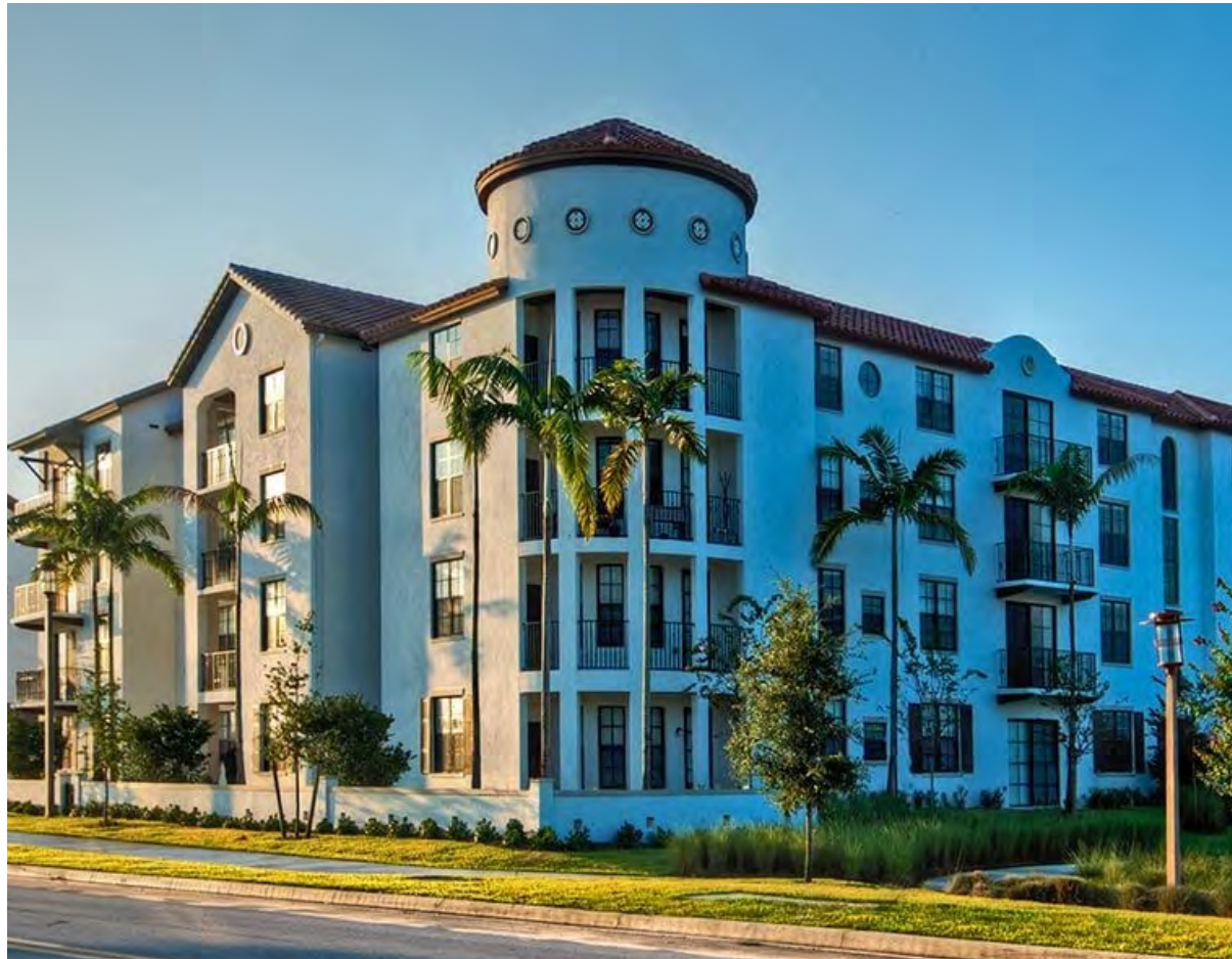
Building corner tower detail
