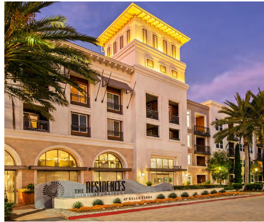
Building corner tower detail & building entrance
